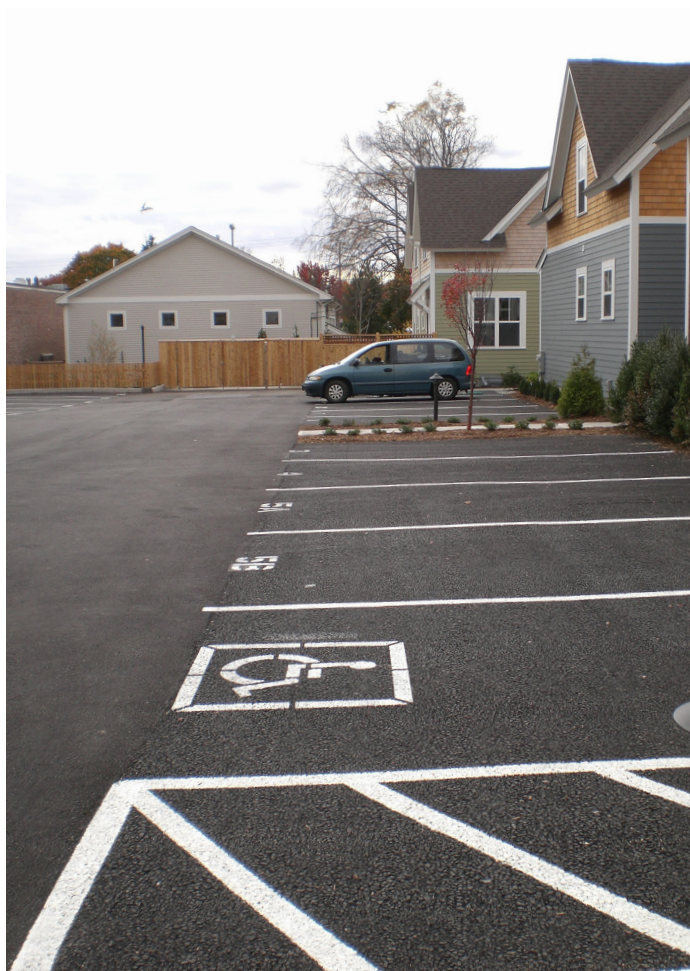
Photo of permeable pavement parking spots at Cottages on the Greene in East Greenwich.
