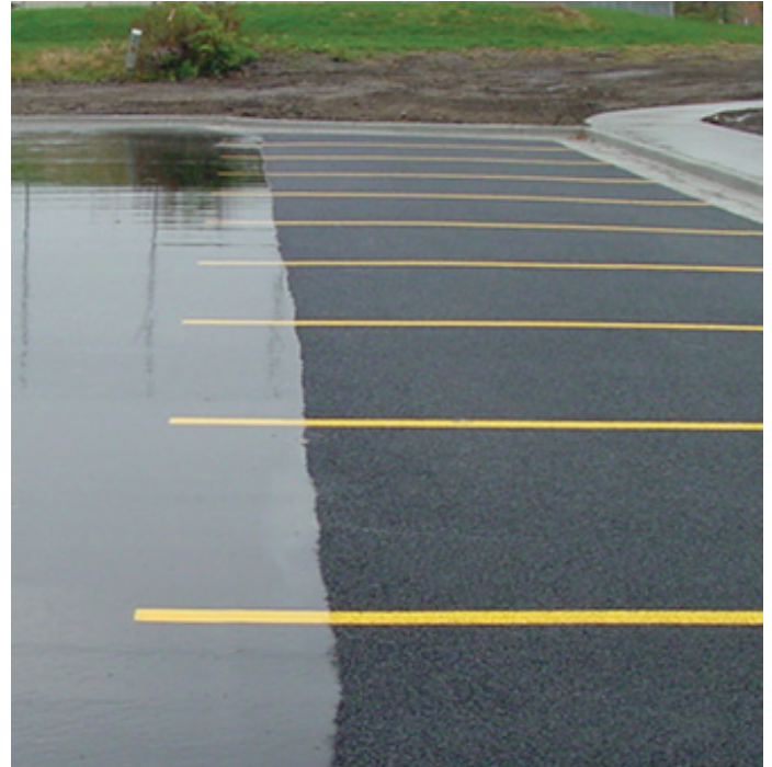
Conventional asphalt on the left, porous asphalt on the right. Photo courtesy of National Asphalt Pavement Association ( www.asphaltpavement.org ).
