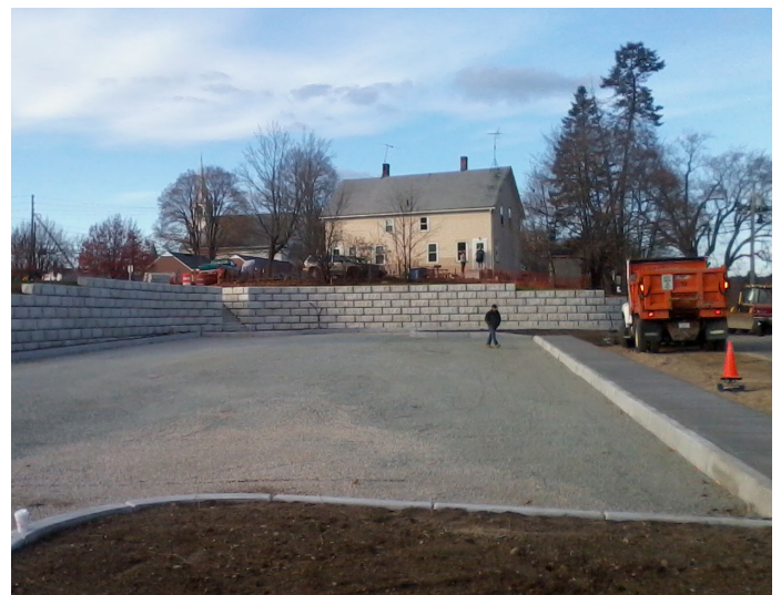
Above, see the base course of stone during the construction of Stillwater Mill auxiliary parking lot in Burrillville. Photo by URI NEMO.
