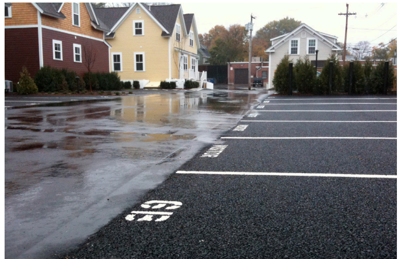
Compare conventional asphalt (left) to porous asphalt (right) during a rainstorm. Photo by Jonathan Ford from Cottages on the Greene in East Greenwich.
