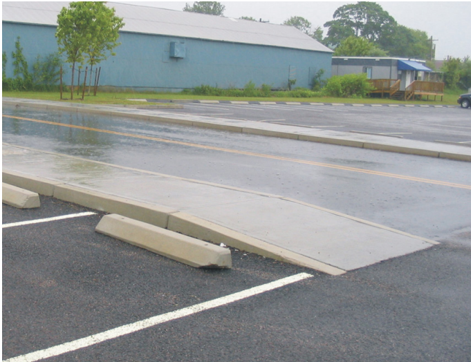
The URI porous asphalt lot in foreground allows rainwater to infiltrate to recharge bed below. The access road beyond is sloped away from the porous asphalt lot and is constructed from conventional asphalt, which will not clog when sediment is deposited by vehicle traffic. Photo by URI NEMO.
