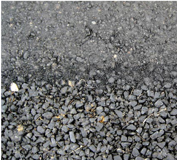
Porous asphalt (bottom of photo) is mixed without fine particles, which allows for the passage of stormwater through the surface. It has a distinct texture when compared to conventional asphalt (top of photo). Photo courtesy of University of Connecticut Cooperative Extension.
