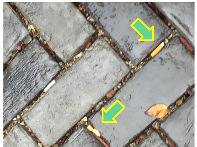
Cigarettes and other small litter may be likely to get caught in the void spaces between block pavers, prompting special maintenance tasks or concerns. Image courtesy of Coastal Green & Resilient Infrastructure Project.
