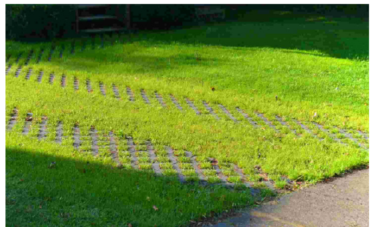
Open-cell design concrete pavers used for a ribbon driveway and walkway. Photo courtesy of the City of Burlington, VT.
