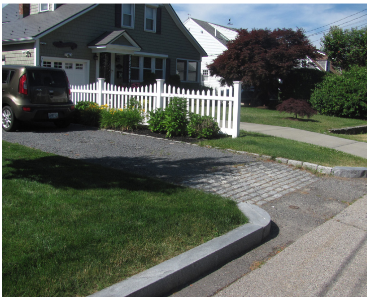
A crushed stone driveway with cobblestone apron and paver border in East Providence.
