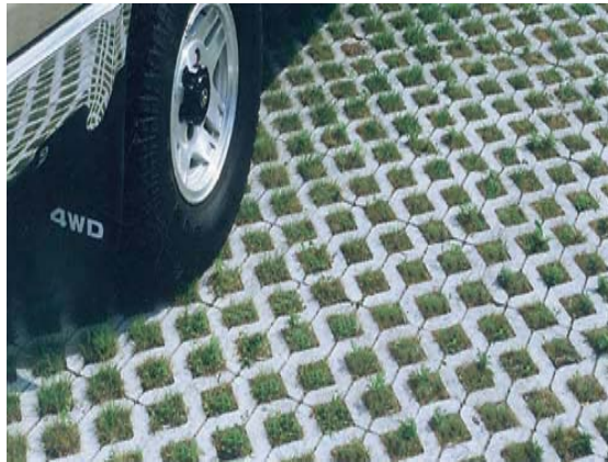
Light duty paver designed for overflow parking, vehicle emergency access
