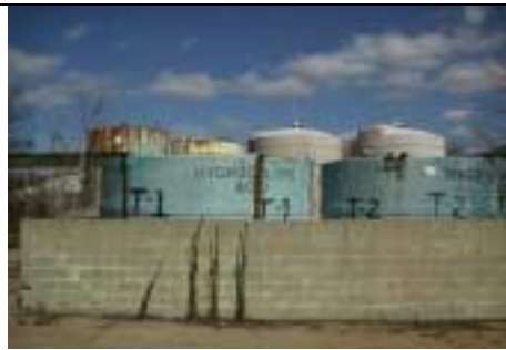
Brownfields and Site Remediation
