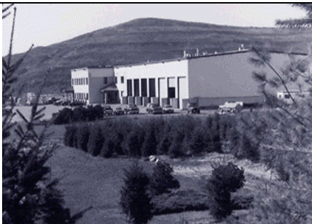
Waste Facility Management
