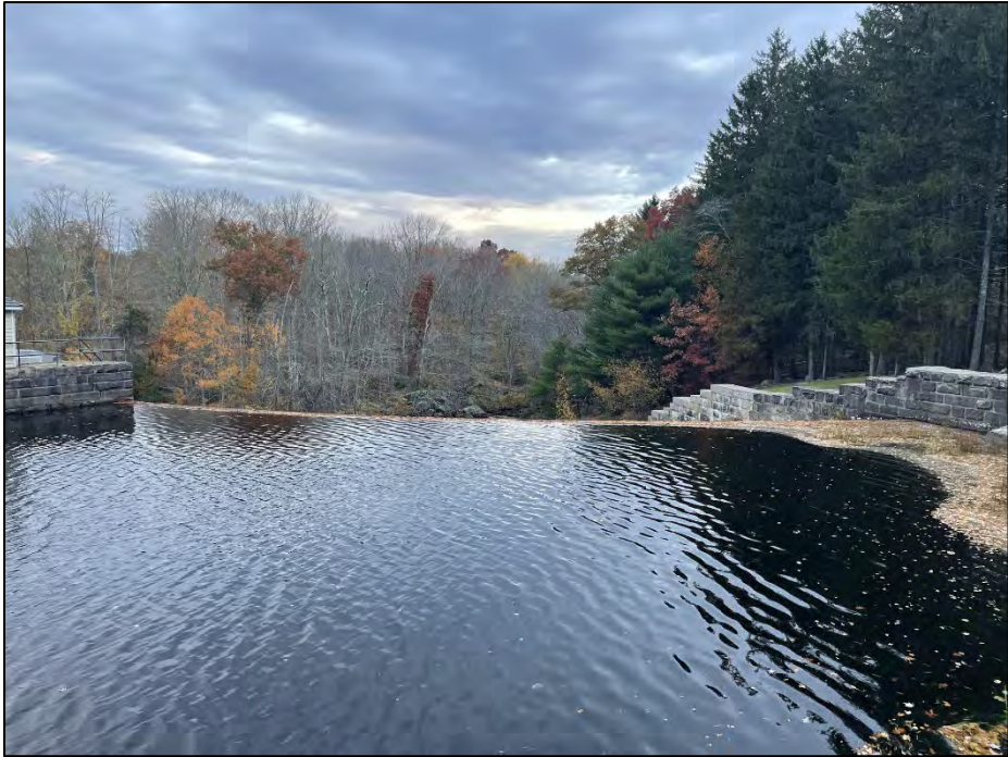
Photo No. 9.: Approach to the spillway looking downstream.
