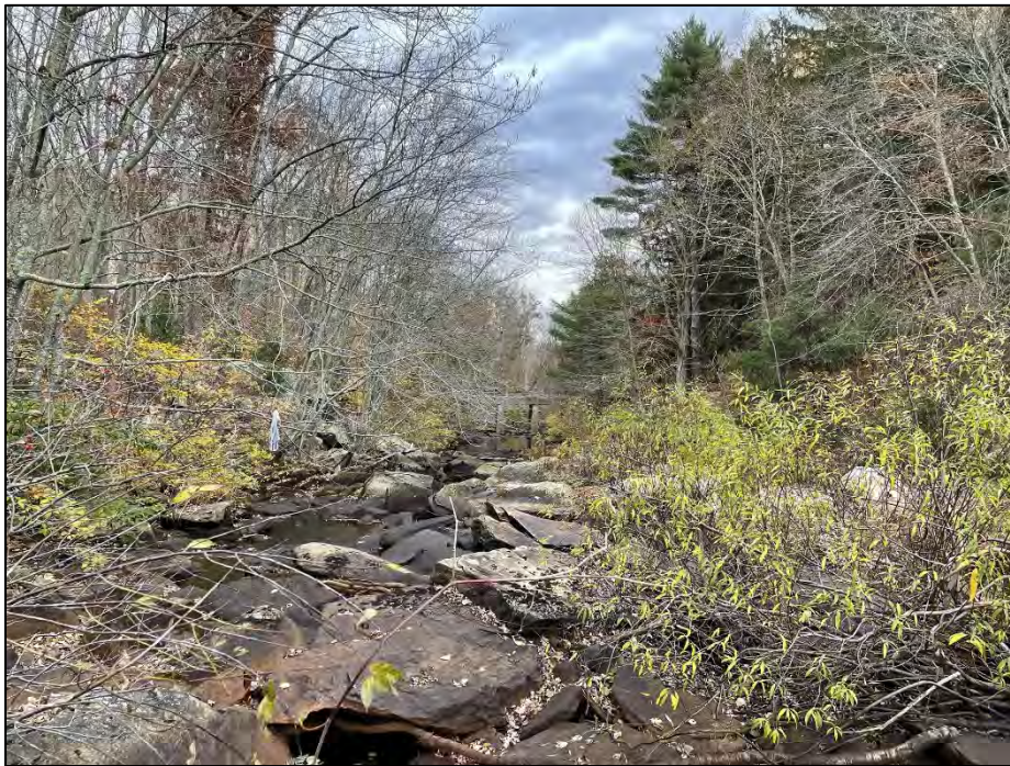
Photo No. 26.: Downstream channel of the spillway from where the "Old Mill Channel" diversion channel converges with the downstream channel of the spillway looking downstream.
