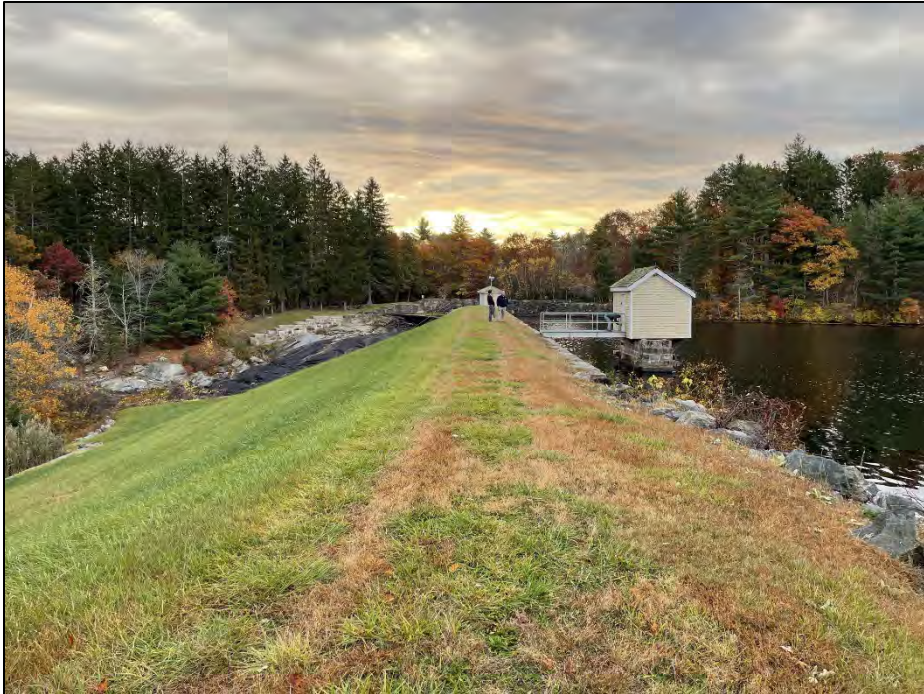
Photo No. 6.: Dam crest from near the left abutment looking right.
