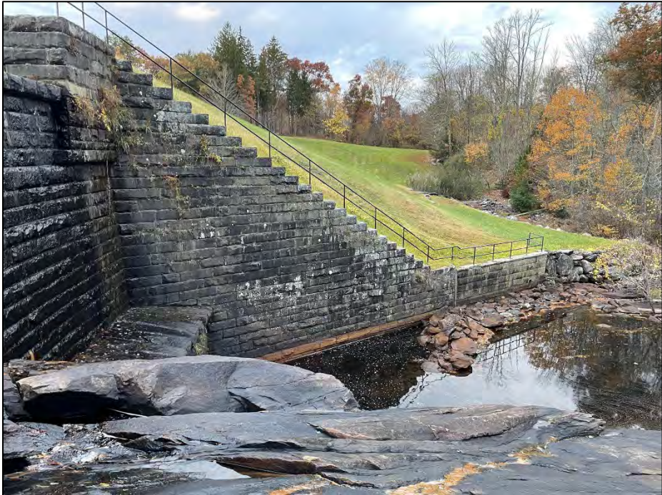
Photo No. 12.: Overview of left downstream training wall of the spillway.
