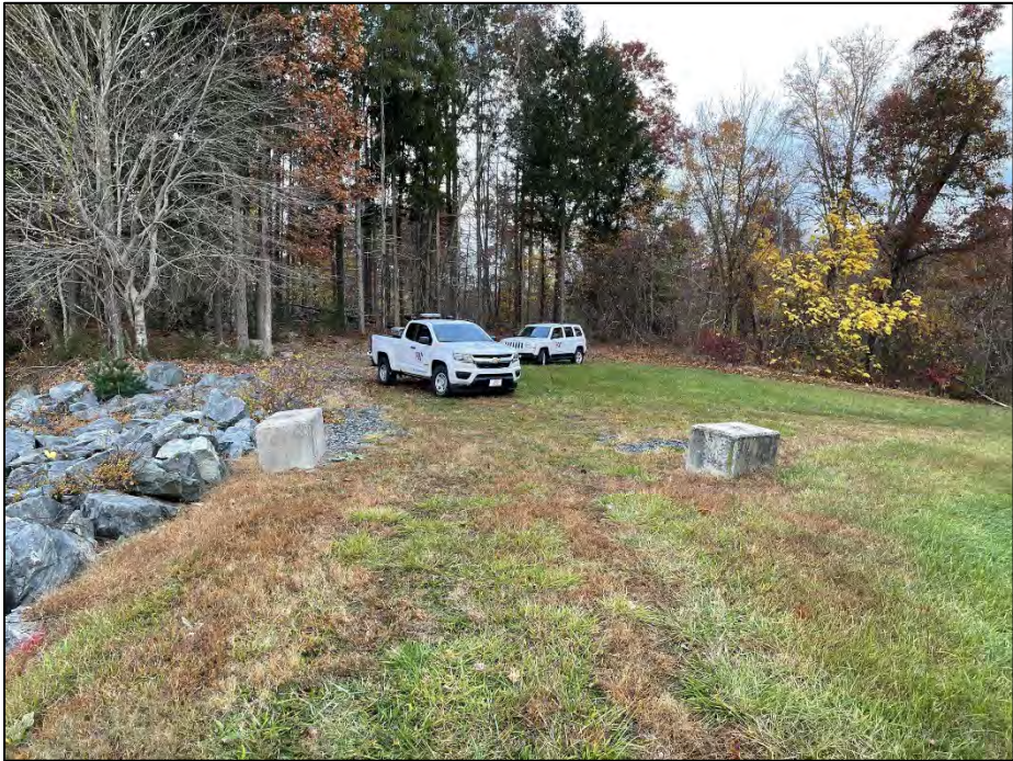
Photo No. 5.: Overview of the left abutment.
