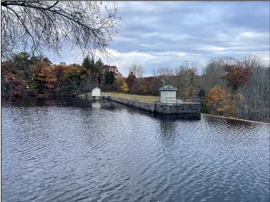
Photo No. 2.: Overview of the dam from the upstream right abutment looking left.
