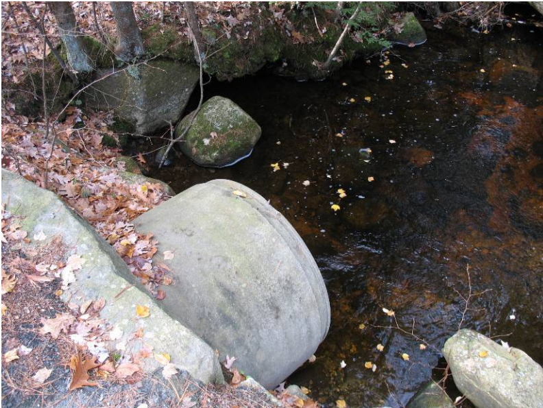
Photo 7: 4-foot diameter pipe under Lakeview Road.
