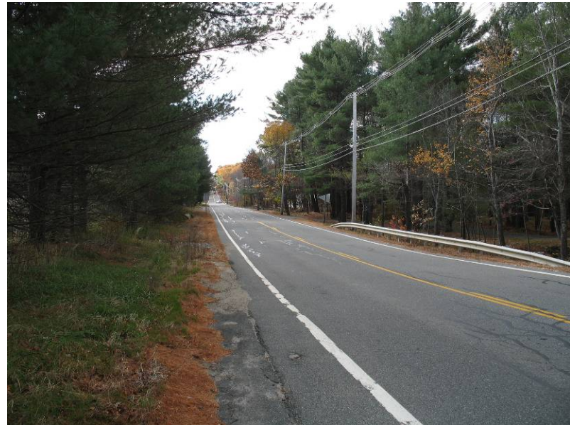
Photo 4: Victory Highway (Route 102) on top of dam.
