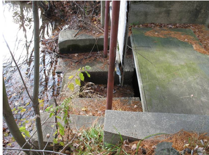
Photo 2: View of spillway from top of dam.
