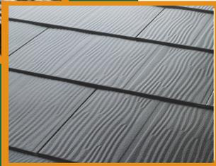
Figure 8: (above right) Class A roofing materials including tile, clay, concrete, slate and asphalt shingles are fire-resistant options. Photo: CSFS
