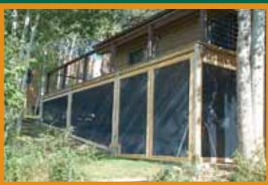
**Figure 15:** *Enclosing decks with metal screens can prevent embers from igniting a house. Photo: Marilyn Brown, La Plata County*
