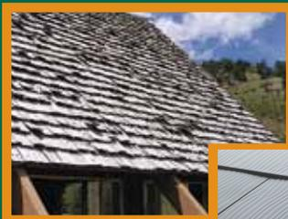
Figure 7: (above) Wood shingle roofs are highly flammable and not recommended. Photo: CSFS
