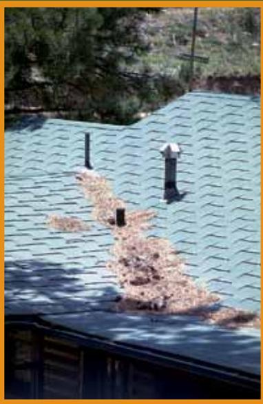
**Figure 14:** *Clearing pine needles and other debris from the roof and gutters is an easy task that should be done at least once a year. Photo: CSFS*
