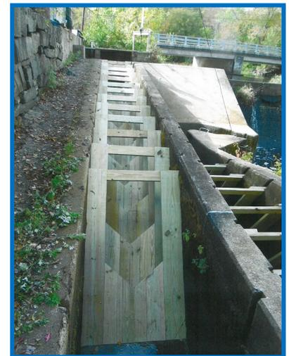
The new fishway baffles decrease water velocity and allow the fish to swim around the obstruction. Photo courtesy of P. Edwards
