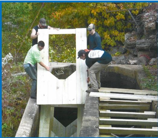
The DFW staff work to install the new Potter Hill Dam fishway baffles. Photo courtesy of P. Edwards
