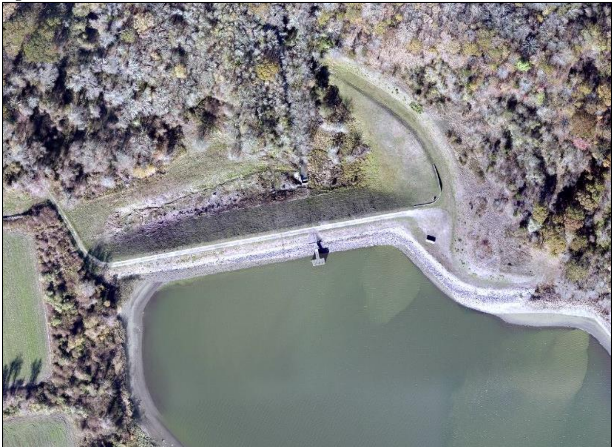
Figure 5.2 Watson Reservoir Dam
