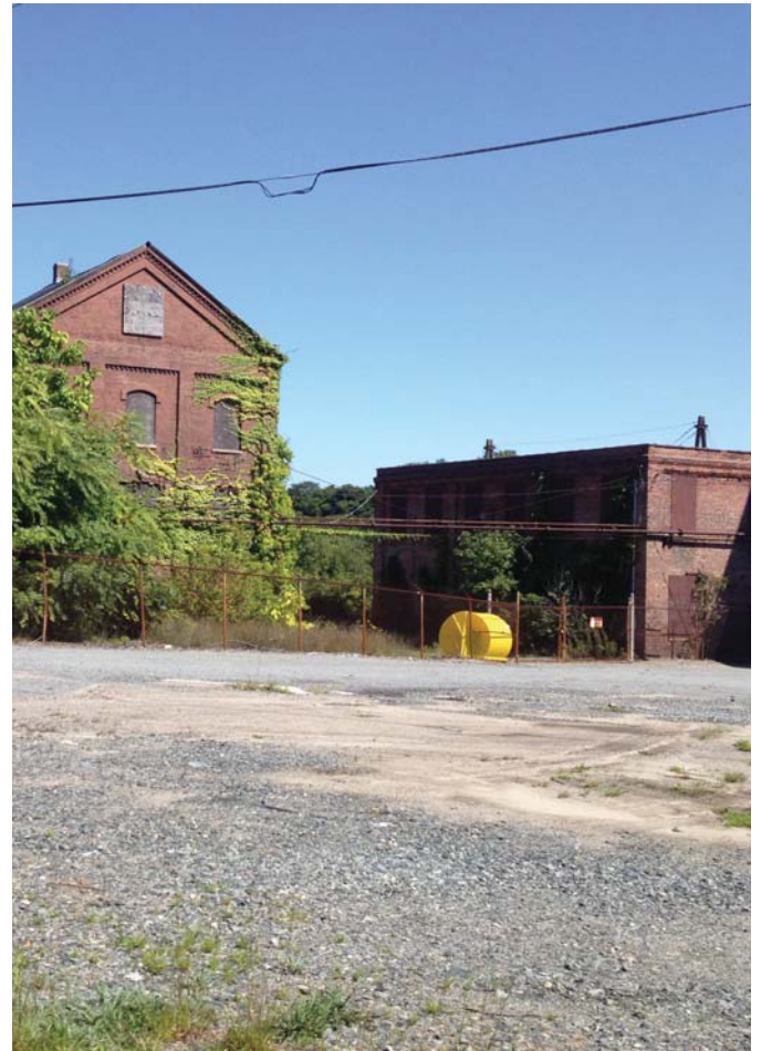
The buildings, which are in a state of disrepair, have been mostly unused since the 1960s.
