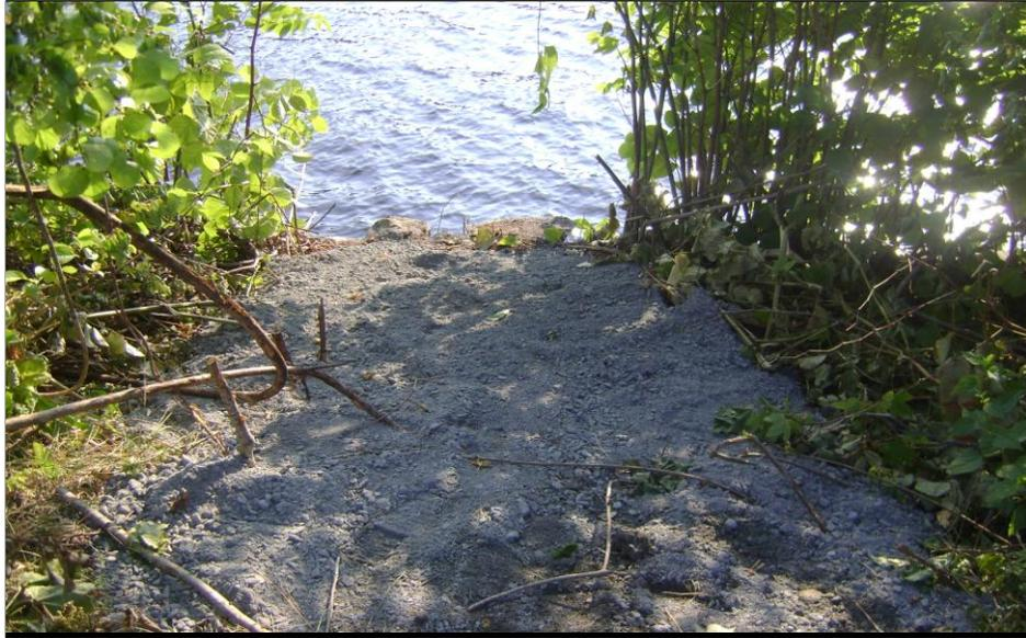
**Crushed stone placement over excavated area and geotextile. August 25, 2011. 8:17 am.**
