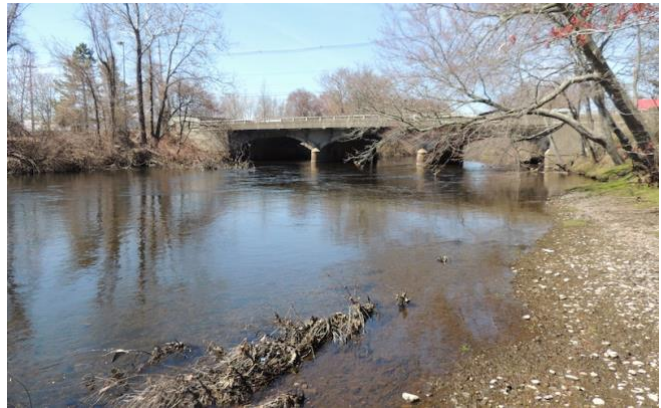
Site of DV-01c at Warwick Ave. bridge looking upriver
