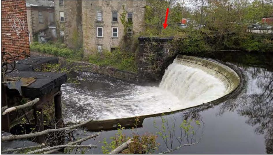
Overview of primary spillway approach and overgrown center embankment (Arrow). – Pare 2019.
