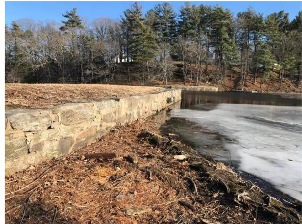
Downstream (left) and upstream (right) sides of the embankment near the left abutment, after removal of improper vegetation, at the Slatersville Middle Dam (No. 046), North Smithfield
