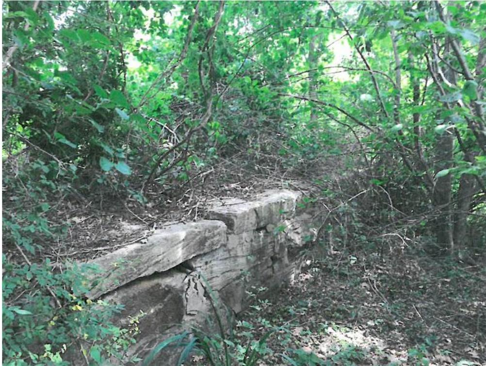
*Overgrown embankment at Slatersville Middle Dam (No. 046) in North Smithfield*
