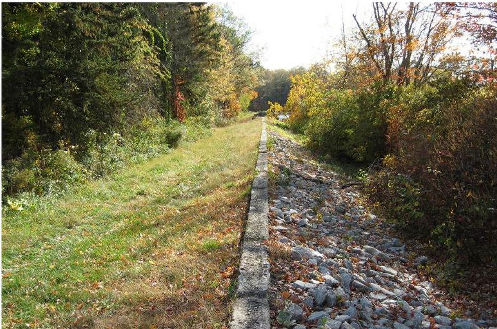
*Improper vegetation on upstream & downstream sides of embankment at Waterman Dam (No. 111) in Gloucester/Smithfield*
