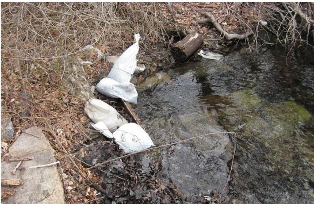
*Sand bags that were apparently used to block flow into the spillway conduit at Creamer Dam (No. 742) in Tiverton*
