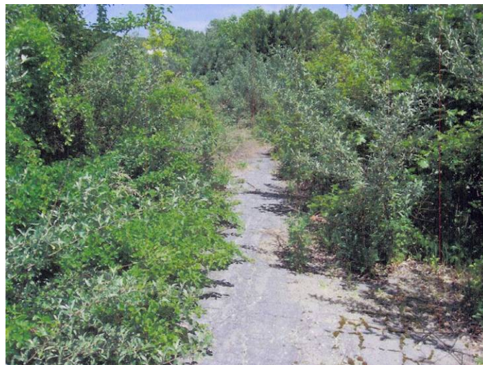
Crest of Stillwater Dam (No. 109) in Smithfield
