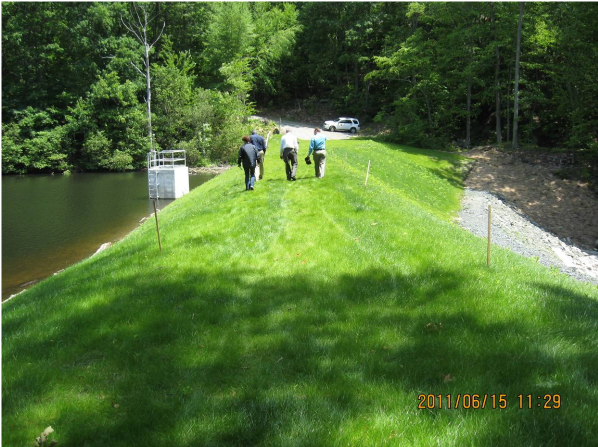
Rehabilitated Limerock Dam (No. 295) in Lincoln
