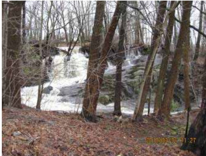
Looking upstream at Clarke's Lower Dam (No. 372) in Cranston
