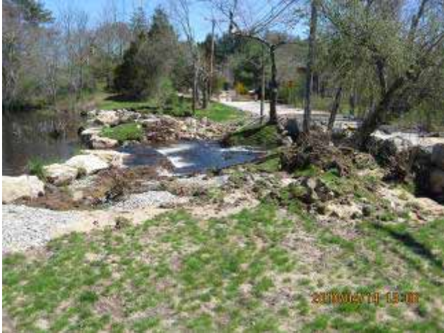
Looking across and upstream at the failed section of Glen Rock Dam (No. 236) in South Kingstown
