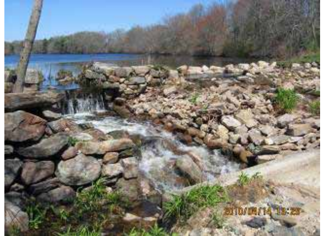
Looking across and upstream at the failed section of Glen Rock Dam (No. 236) in South Kingstown
