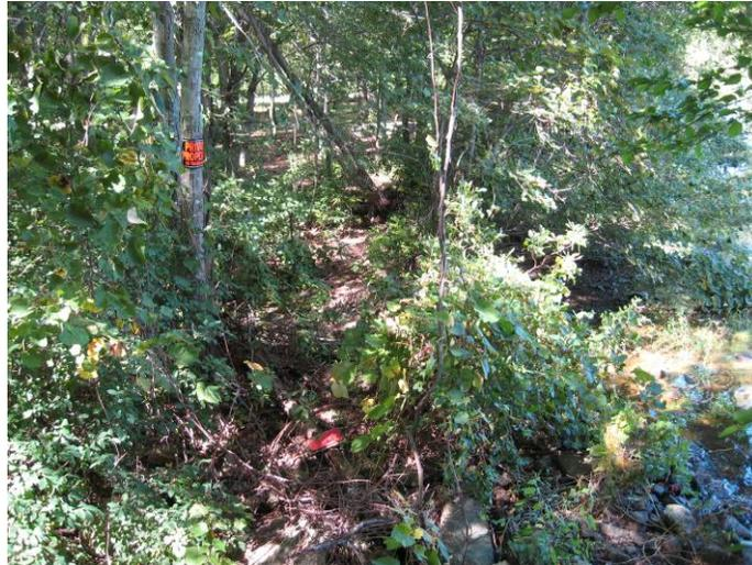
Improperly vegetated spillway at Almy Dam (No. 169), Johnston
