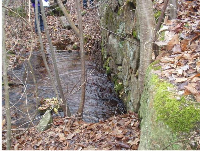
Seepage/leakage at Blue Dam (No. 229), Hopkinton
