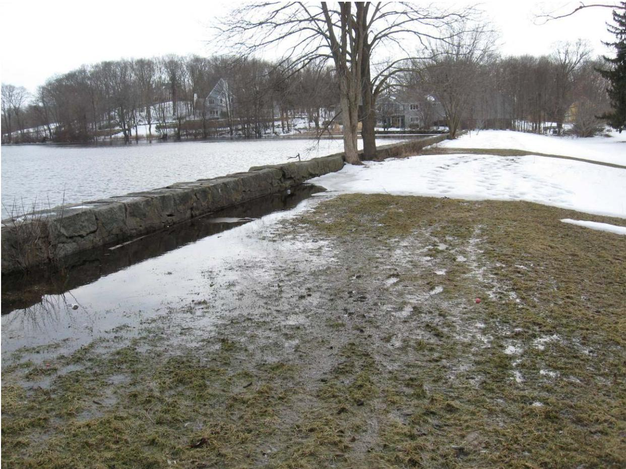
Overtopping earthen embankment of Creamer Dam (No. 742), Tiverton
