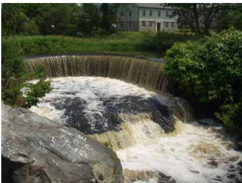
Spillway at Horseshoe Falls Dam (No. 249), Charlestown/Richmond
