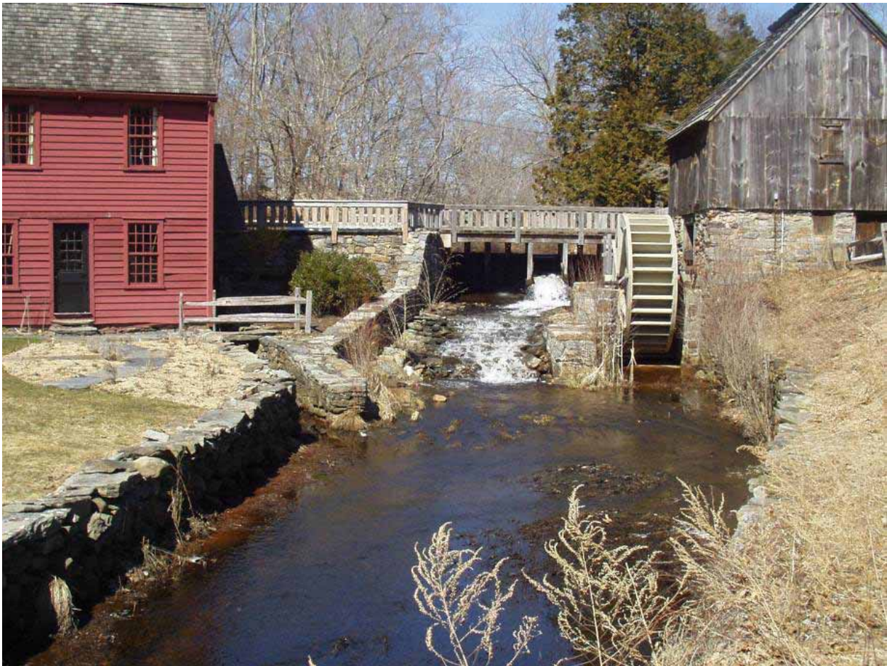
Spillway at Gilbert Stuart Pond Dam (No. 513), North Kingstown
