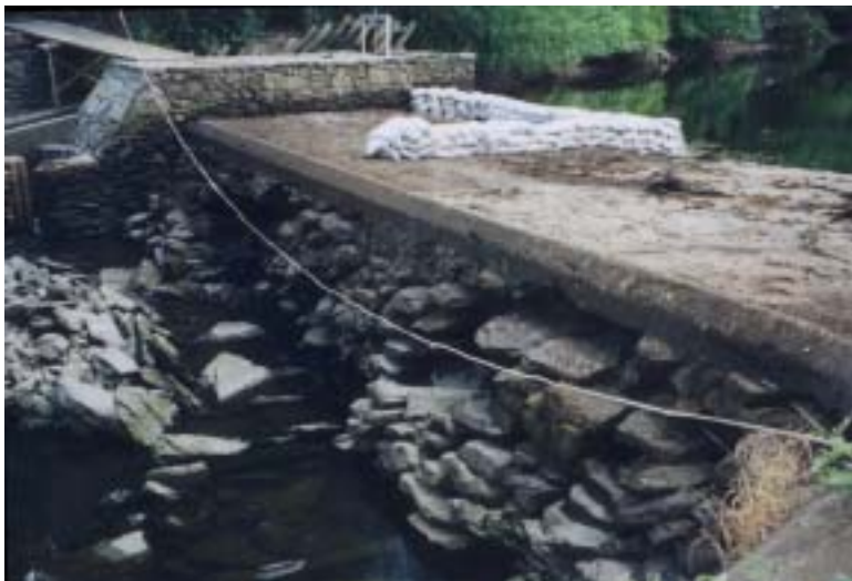
Dam Number 296 (Old Forge Mill), North Kingstown
