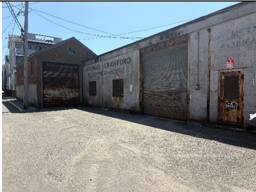
View of temporary cap area.
