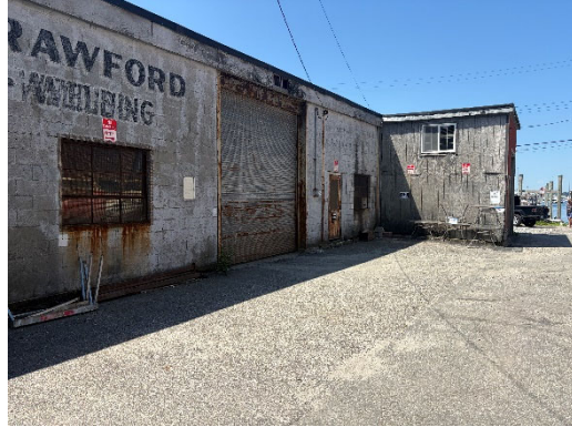
View of temporary cap area.
