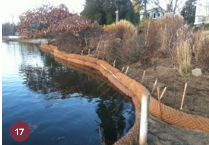
Coir Log Coir fiber logs comprised of natural fibers are key component of stabilizing and replanting eroded areas. Staked and layered with live ‘whips’ of native plants, the coir fiber logs help hold the soil as they slowly decompose.
