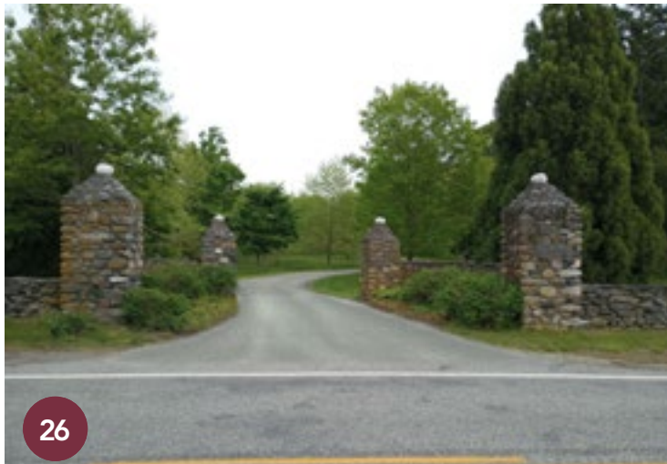
Stone Columns and Walls Field stone walls exist on the site in several locations. Repairing the walls and in some areas constructing new stone walls to define spaces is recommended. Formalizing the entrance to the Park with stone columns or similar treatment allows for installation of an entrance gate and will create an enhanced sense of arrival.
