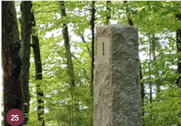
Trail Marker Durable posts made of granite are in use in other state parks. They are highly resistant to vandalism and require little maintenance. Text may be a panel that is then affixed to the post, or the markings may be engraved as shown above.
