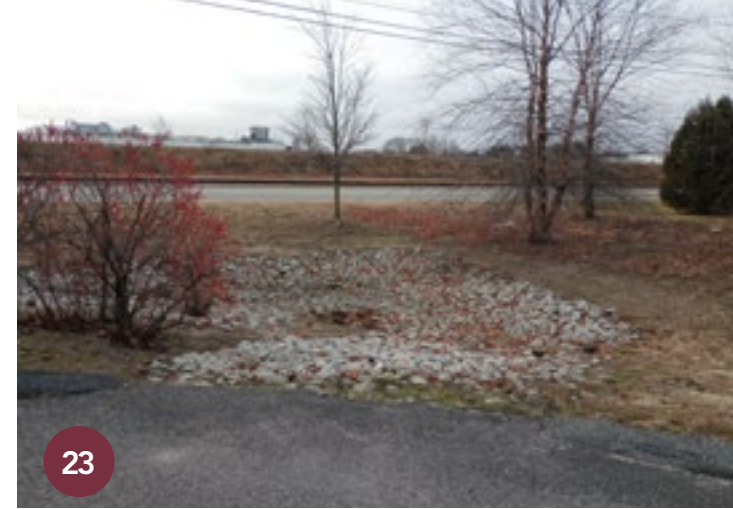
Rip Rap-Lined Swale Stone lined swales may be utilized in areas with higher volumes of water. Irregular edges plated with native plants is desirable. Voids in the rip rap may be planted to further visually soften the appearance and attenuate flow.
