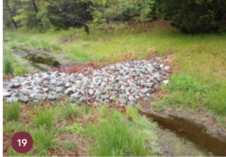
Check Dam Stone check dams incorporated into high volume swale systems will slow and attenuate stormwater flow. Use of stone slabs or naturally occurring, weathered stone bedded and flanked with smaller round stone is visually preferred to the use of crushed rip-rap in this park setting.
