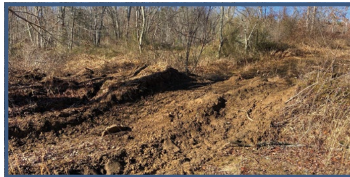
If slope, grade, and drainage are not taken into account, severe erosion and road damage can occur.
