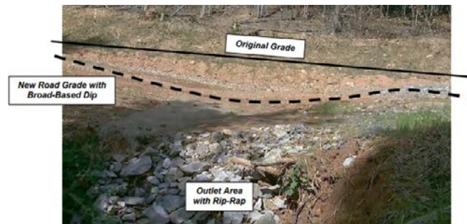
Figure 5A: Cross-section view of a broad-based dip and outlet
