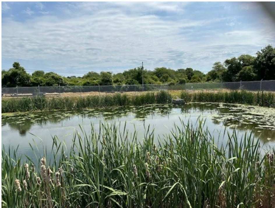
Installation of green stormwater infrastructure functions to mitigate multiple pollutants (sediment, nutrients, bacteria) from previously untreated agricultural runoff on a farm in Middletown, Rhode Island.
