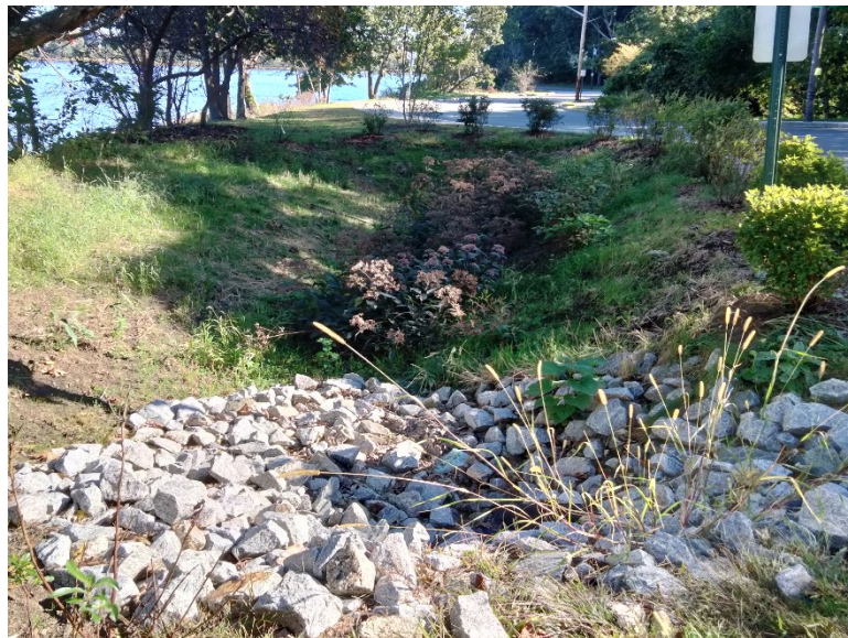
Installation of green stormwater infrastructure to mitigate multiple pollutants (sediment, nutrients, bacteria) along the Seekonk River in Providence.
