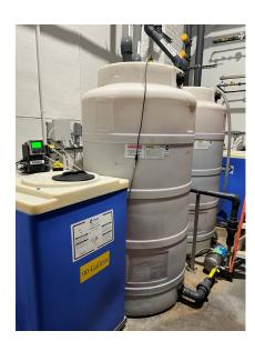
Our well water feeds through green sand filters and is pH and chlorine adjusted on the way to the Cold Water Tank ☐ Hot water tank
