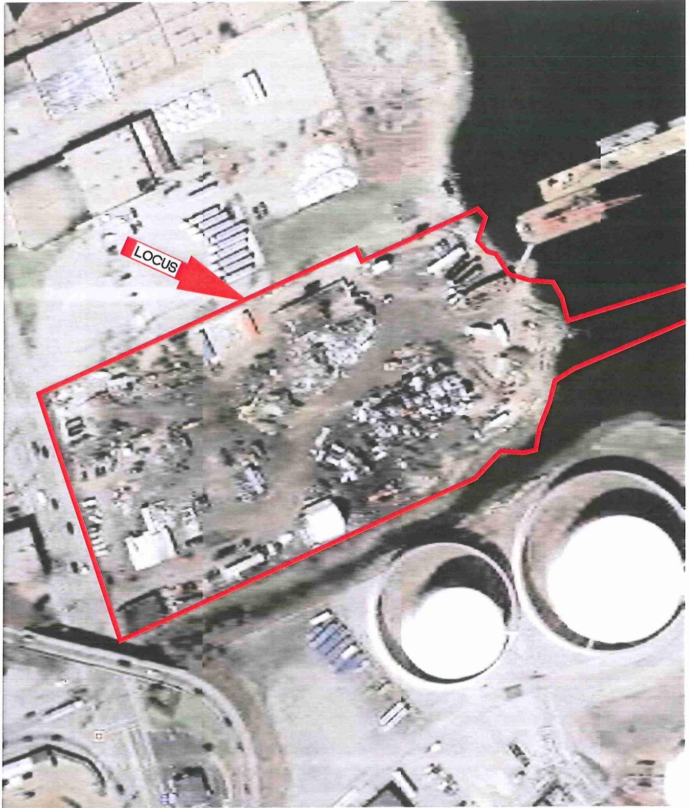
AERIAL PHOTO OF PROPOSED CONSTRUCTION SITE
