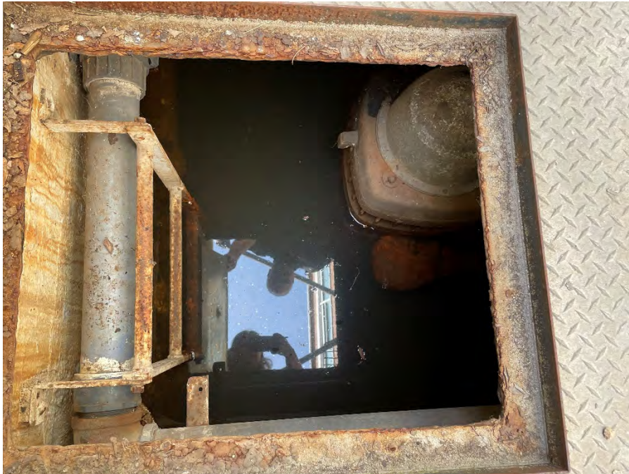
Interior of Vault with Sub-Grade Relic Infrastructure
