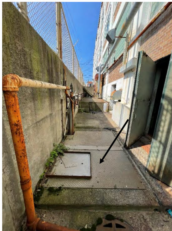
Vault with Sub-Grade Relic Infrastructure
