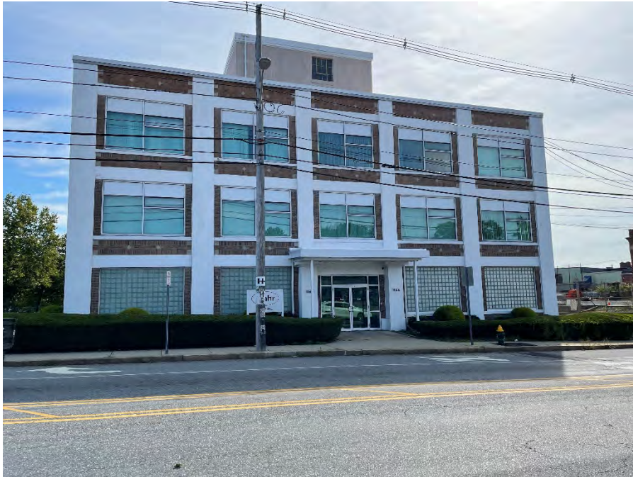
Representative View of the West Side of the Site Building (looking east)
