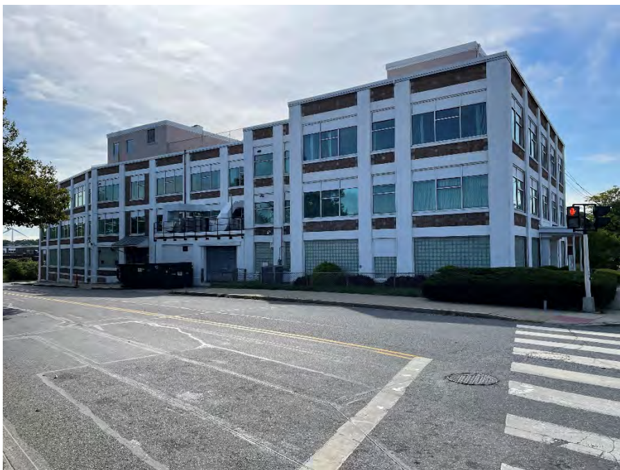
Representative View of the North Side of the Site Building (looking south)
