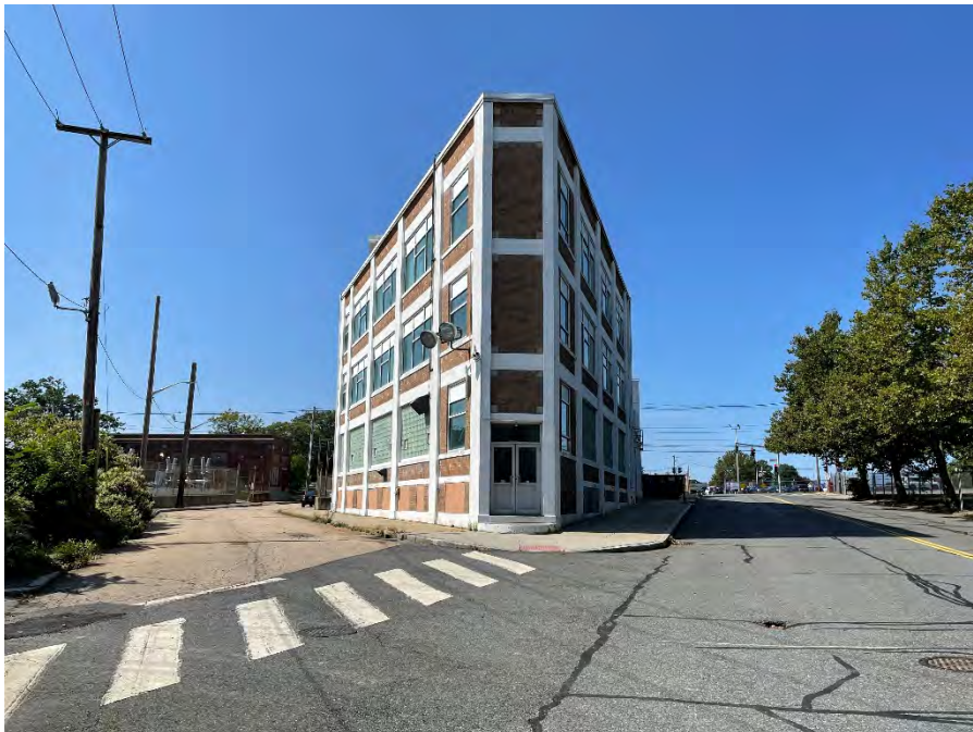
Representative View of the East Side of the Site Building (looking west)
