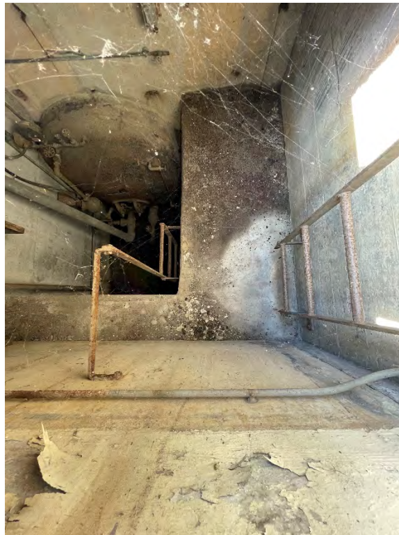
Interior of Sub-Grade Vault
