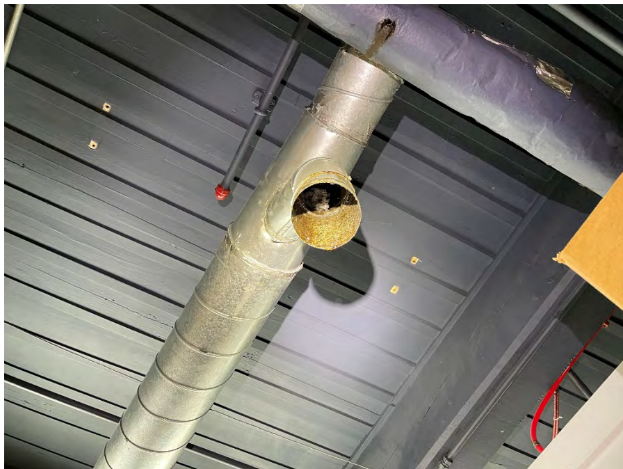
Relic Vent – Reportedly Utilized to Filter Dust and Particulates
