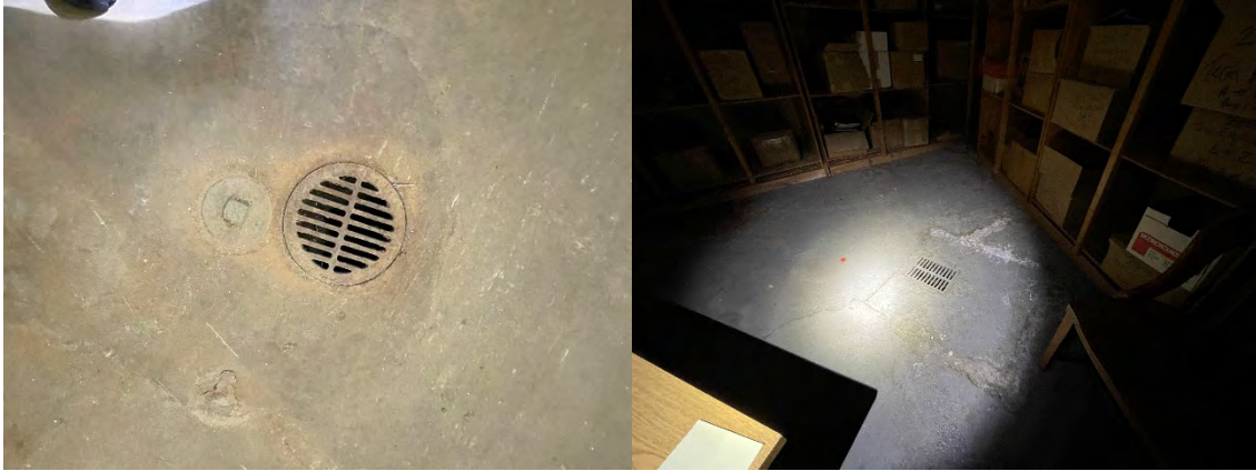
Representative View of Floor Drains – Basement
