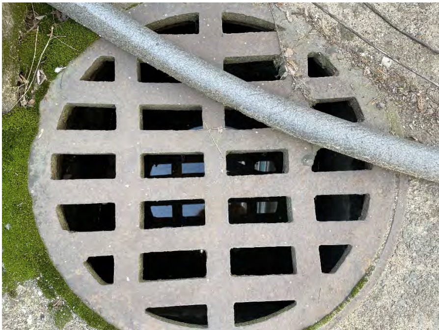
Representative View of Drainage Structure – South Side of Building – Fenced-In Area
