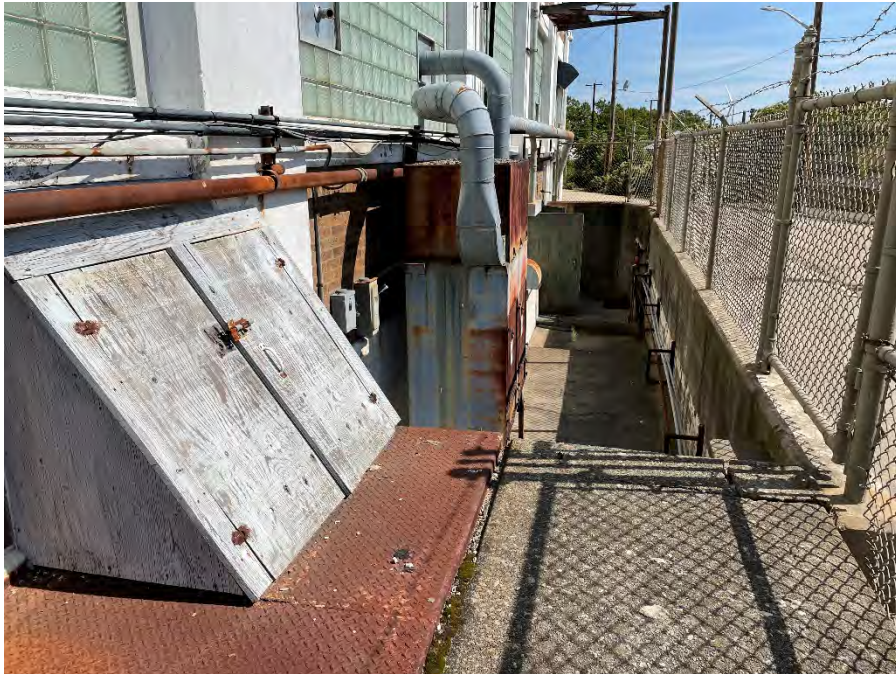
Wooden Bulkhead – Access to Sub-Grade Vault
