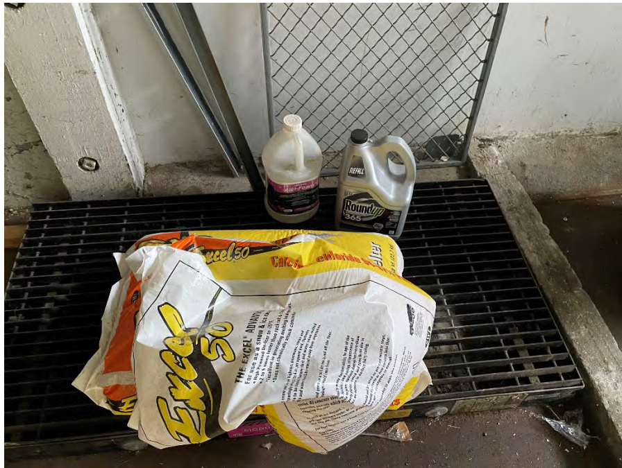
Spill Containment Structure
