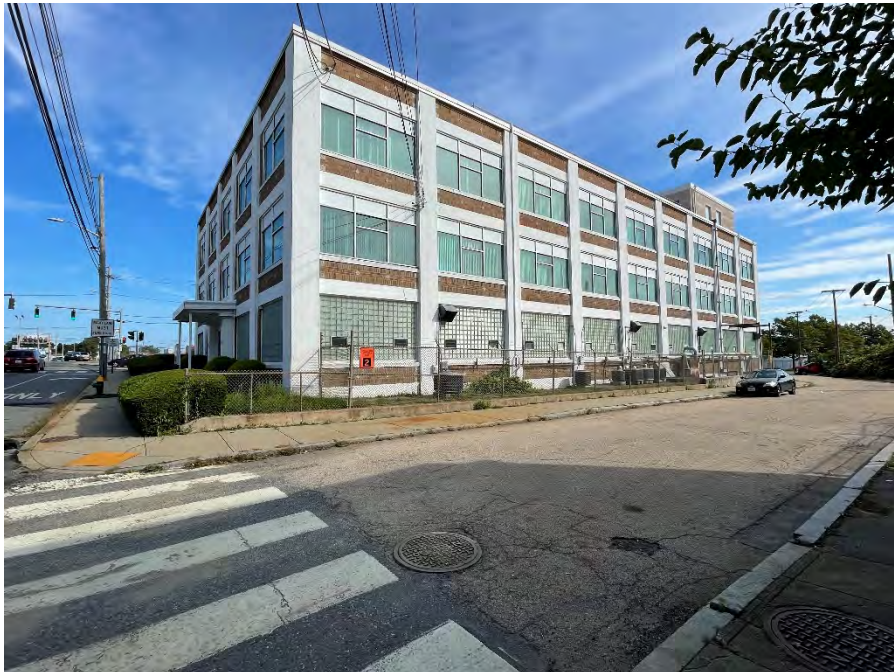
Representative View of the South Side of the Site Building (looking north)
