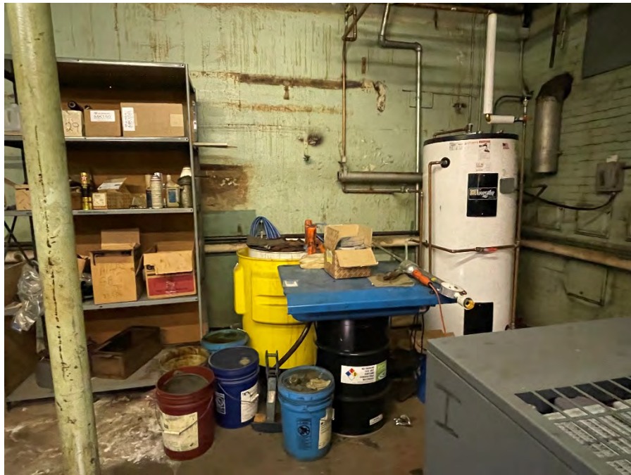
Five (5)-gallon Plastic Buckets with Varying Quantities of OHM Parts Washer-degreaser and Associated 55-gallon Steel Drum in an Overpack Drum (Blaser Swisslube).
