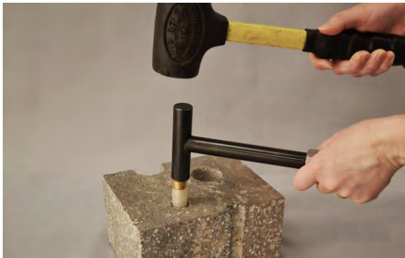
Figure 2. Installing the VAPOR PIN®
