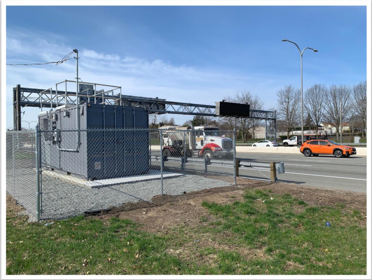
Figure 13: New Cranston Near-Road Monitoring Location (facing SW)
