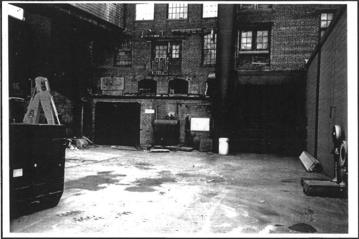
Photo No. 3: View of 275-gallon AST No. 6 overflow tank in the courtyard area to the north of Building 6.
