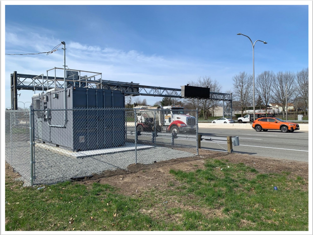
Figure 13: New Cranston Near-Road Monitoring Location (facing SW)
