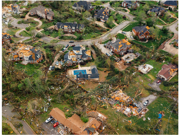
Hurricane Damage in Florida
