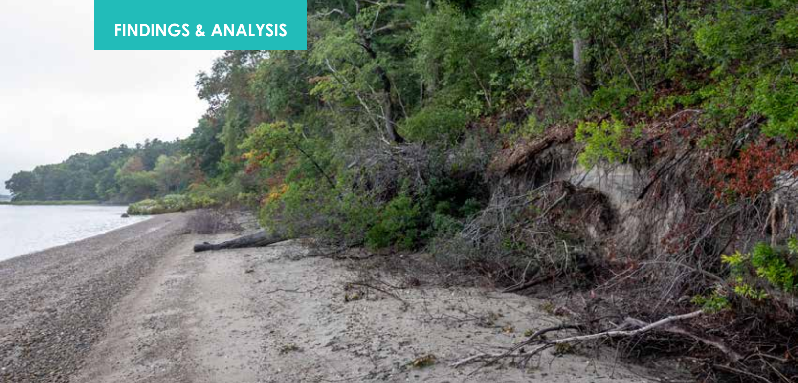
Erosion damage at Goddard Memorial State Park
