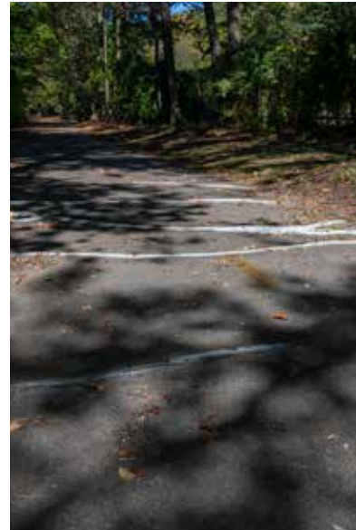
White paint highlights root damage to the Blackstone Valley Bike Path
