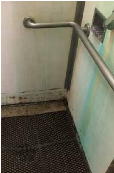
Example of an aging infrastructure at Burlingame State Park Campground
