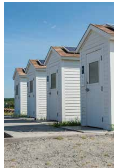
Bathroom facilities at East Beach in Charlestown
