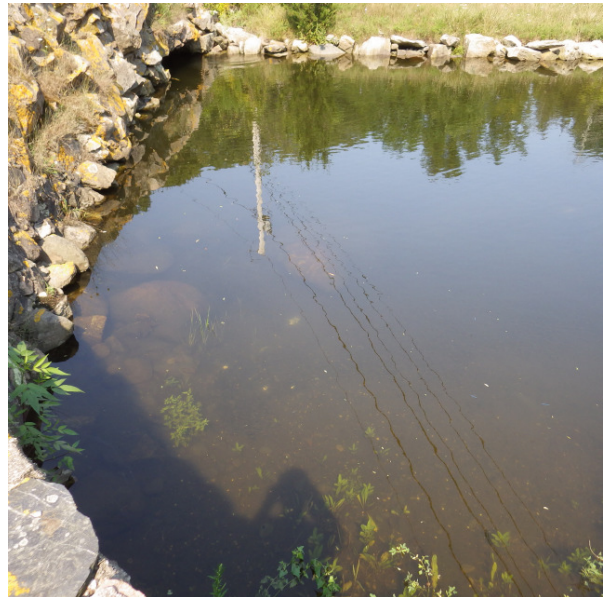
Fig. 4. Sta 3 looking towards small culvert between Sin & Flesh brook and the Gut
