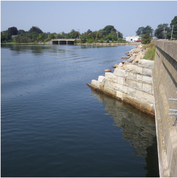
Fig. 1. Tidal culvert opening on Main Rd at Sta 1 between the Gut and northern end of Nanaquaket Pond , looking SW towards Nannaquaket Rd bridge.
