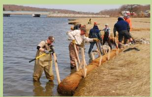
Shoreline erosion prevention using coconut fiber coir logs and recycled oyster shells at the John H. Chaffee NWR, Narragansett, RI. Source: TNC 2014
