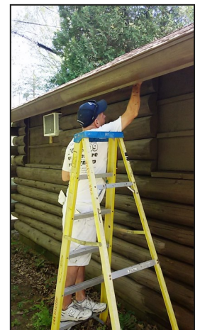
Volunteer, Brian, puts a fresh coat of paint on a Great Swamp cabin.
