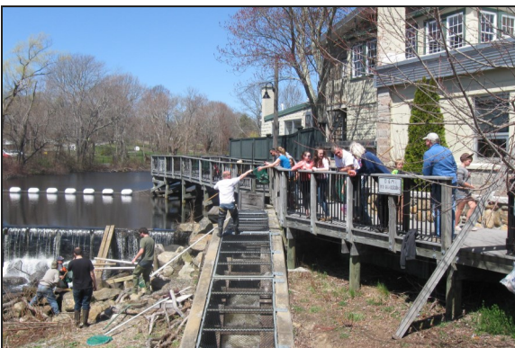
Volunteers & staff working together to lift river herring over the Main St., Wakefield dam, before the completion of the successful fish ladder renovation this year.
