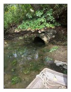
Source 2017-16-118 is a 24-inch Reinforced Concrete Pipe running under the East Bay Bike Path. The source was sampled on 9/14/2017 as the tide was coming in so the flow could not be accurately measured and the elevated bacteria count of 4000 CFU/100ml may be inaccurate due to the tidal influence. The source was not revisited because it is located within the prohibited waters of Bullocks Cove, which will not be reclassified due to the number of marinas within the cove.
