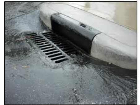
Stormwater runoff entering a storm drain
