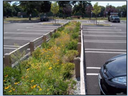
Bio-retention inlet for stormwater runoff from the parking lot at Bristol Town Beach
