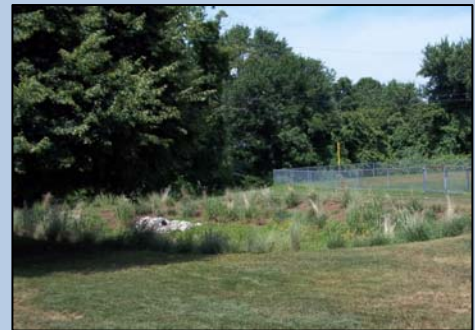
Vegetative infiltration basin at Bristol Town Beach
