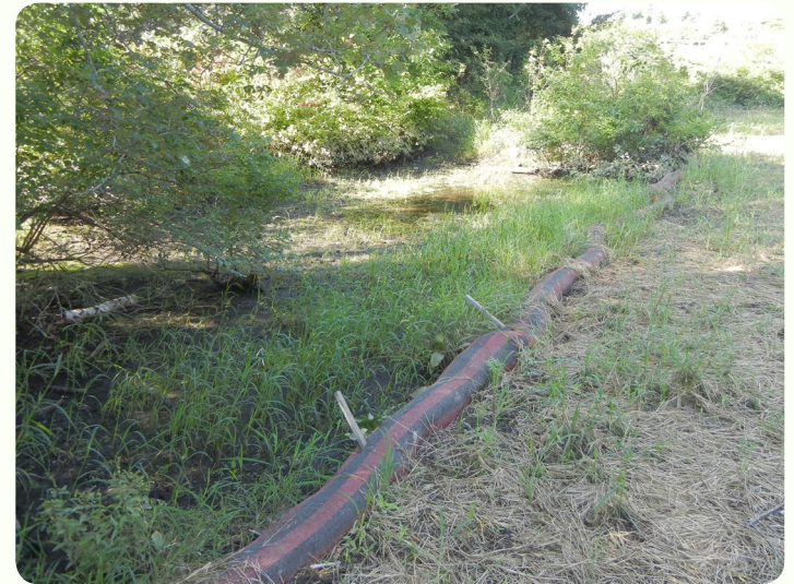
LEFT: Dumpster properly covered with ends weighted down. CENTER: Sediment control blankets can be installed on slopes to prevent erosion before turf is established. RIGHT: Filter socks should be installed between construction and natural resources as shown with the wetland area above (RIDEM).
