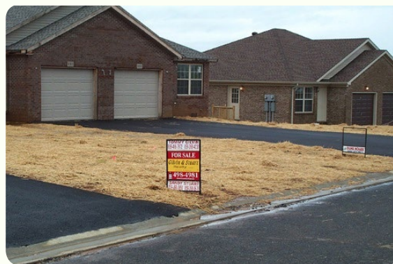
LEFT: Sediment from this construction site has washed across the road, into the storm drain, and then directly into the bay. CENTER: Simply covering bare soil with a thick layer of straw mulch can dramatically reduce erosion (Tetra Tech). RIGHT: This storm drain cover is stopping sediment before it can enter the catch basin (US EPA).
