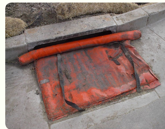
LEFT: Sediment from this construction site has washed across the road, into the storm drain, and then directly into the bay. CENTER: Simply covering bare soil with a thick layer of straw mulch can dramatically reduce erosion (Tetra Tech). RIGHT: This storm drain cover is stopping sediment before it can enter the catch basin (US EPA).
