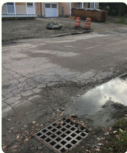
LEFT: Sediment from this construction site has washed across the road, into the storm drain, and then directly into the bay. CENTER: Simply covering bare soil with a thick layer of straw mulch can dramatically reduce erosion (Tetra Tech). RIGHT: This storm drain cover is stopping sediment before it can enter the catch basin (US EPA).
