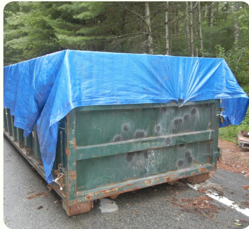
LEFT: Dumpster properly covered with ends weighted down. CENTER: Sediment control blankets can be installed on slopes to prevent erosion before turf is established. RIGHT: Filter socks should be installed between construction and natural resources as shown with the wetland area above (RIDEM).
