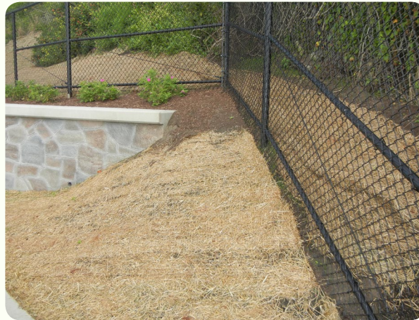
LEFT: Dumpster properly covered with ends weighted down. CENTER: Sediment control blankets can be installed on slopes to prevent erosion before turf is established. RIGHT: Filter socks should be installed between construction and natural resources as shown with the wetland area above (RIDEM).
