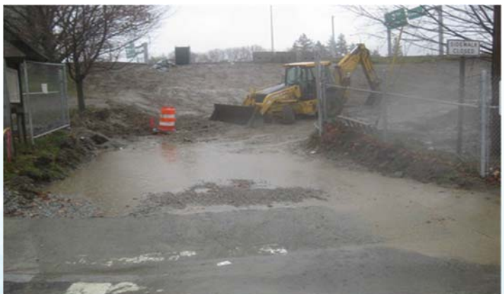
A non-compliant RIDOT construction site
