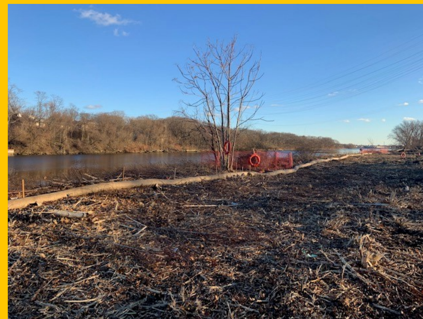
Straw Wattles Limit Erosion
