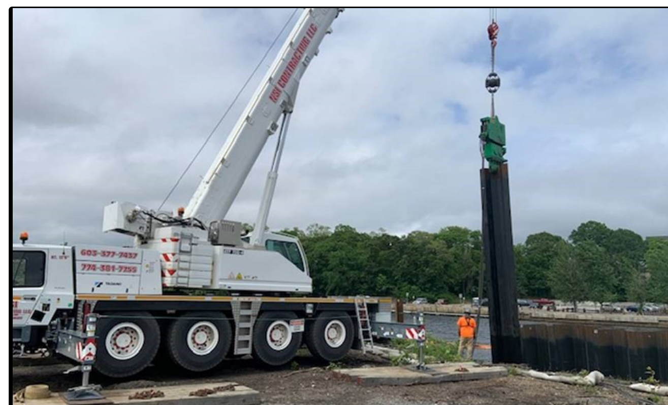
Construction of Barrier Wall - Sheet Pile Installation
