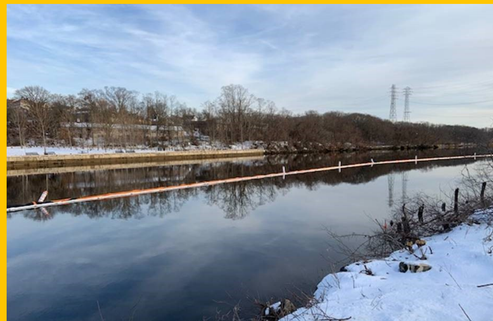
Turbidity Curtains Prevent Sediments From Migrating Away From Site
