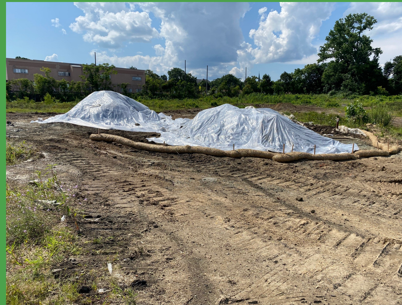
Covered Stockpiles Control Dust and Odors
