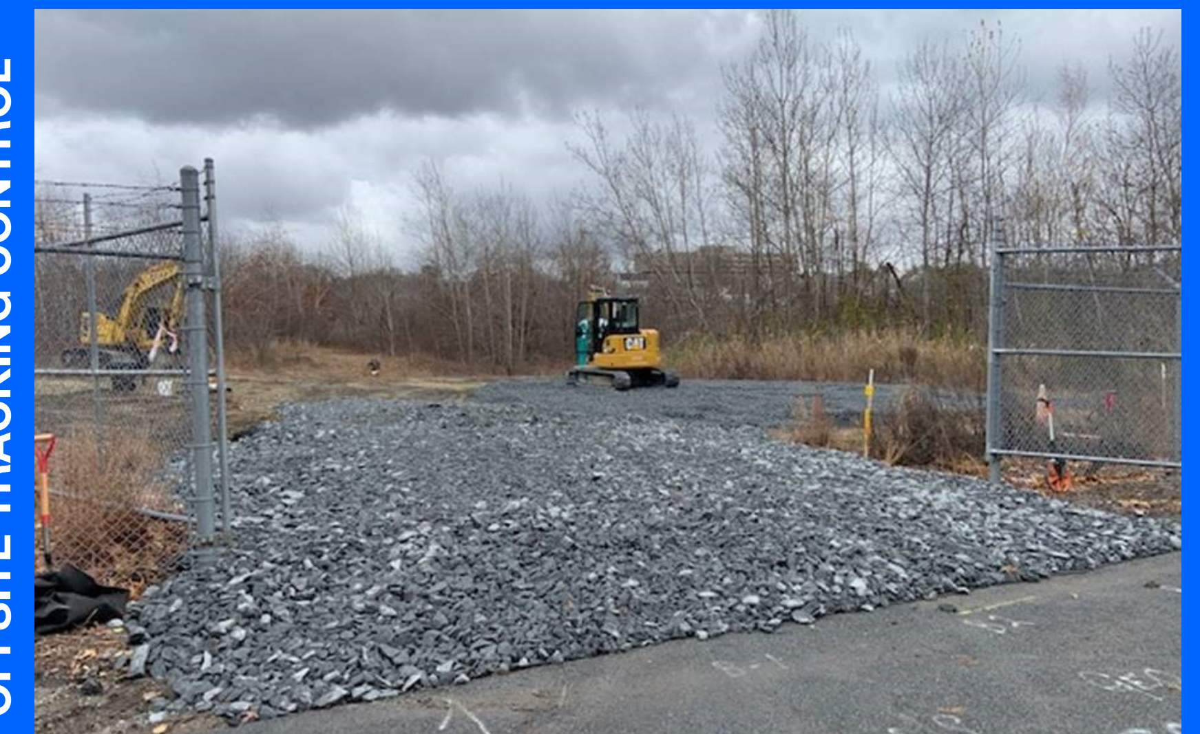
Tracking Pad Prevents Offsite Tracking of Material
