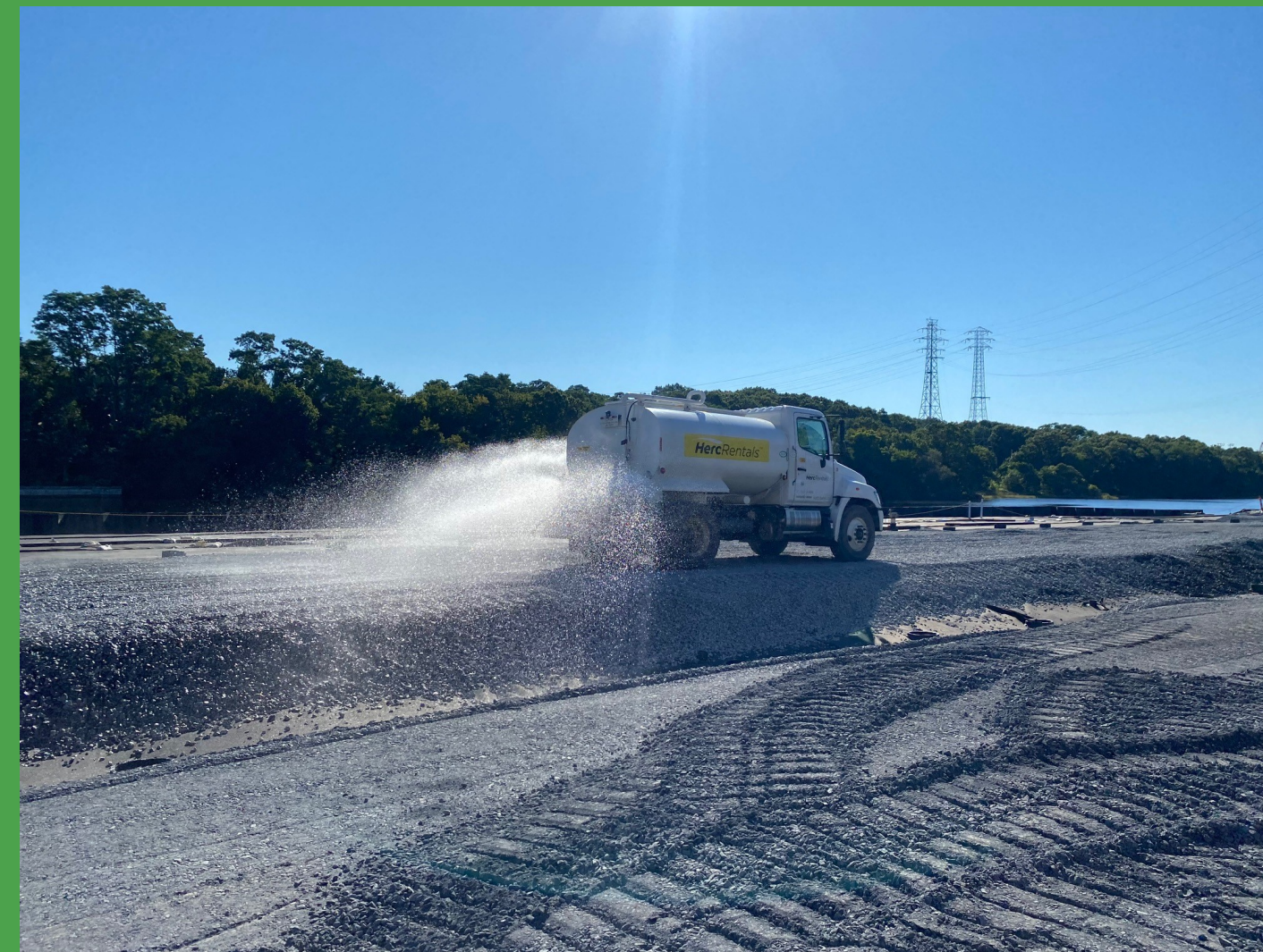
Water Truck Control Dust
