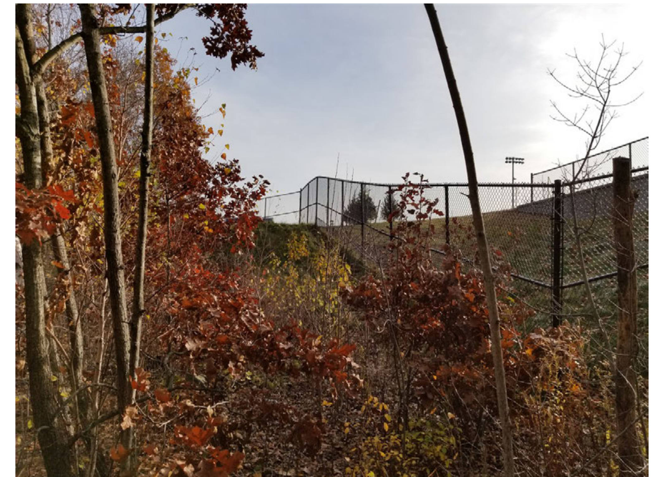
Chain Link Fencing Southwest Portion of the Site
