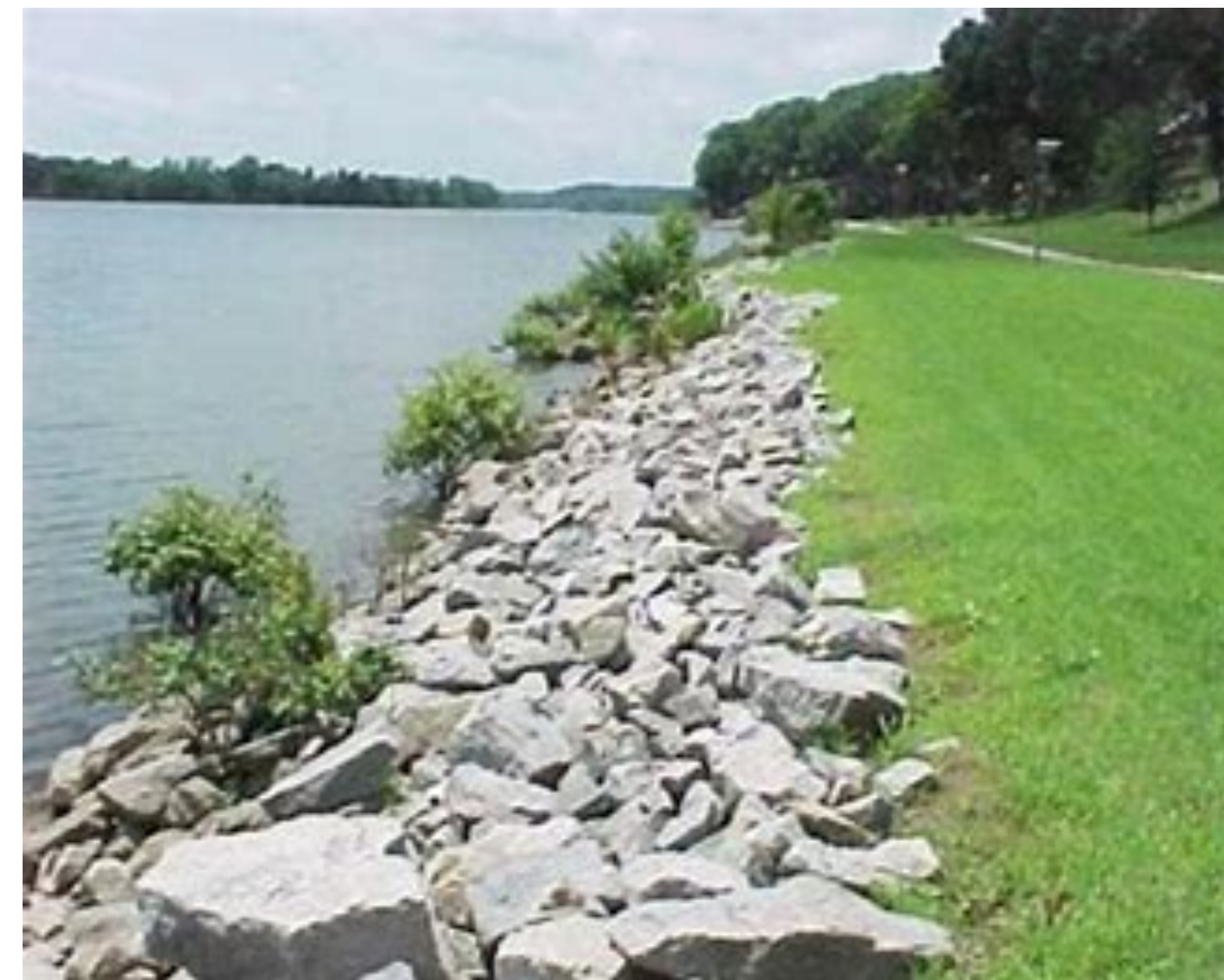
Example of a Riprap Revetment
