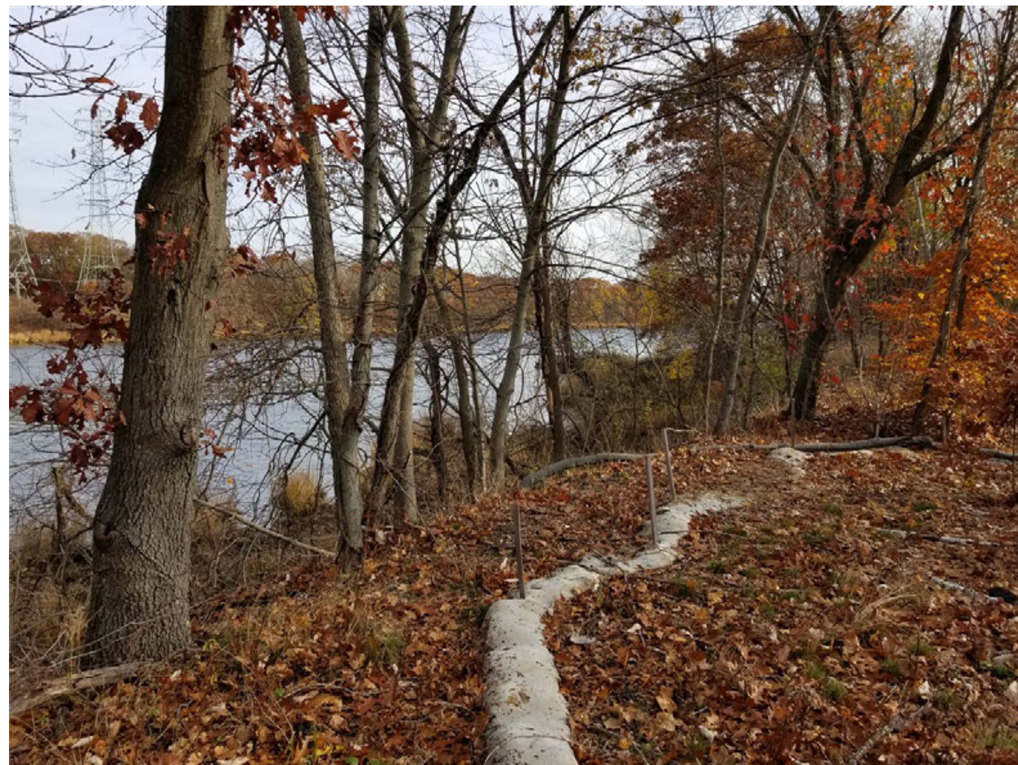
Manmade Earthen Riverbank Southern Portion of the Site
