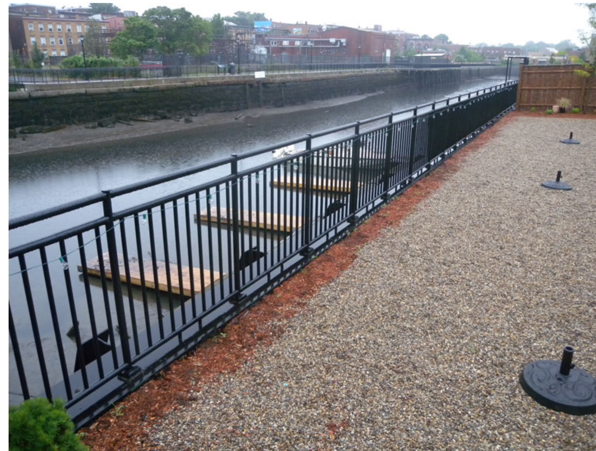
Example of Bulkhead Railing System
