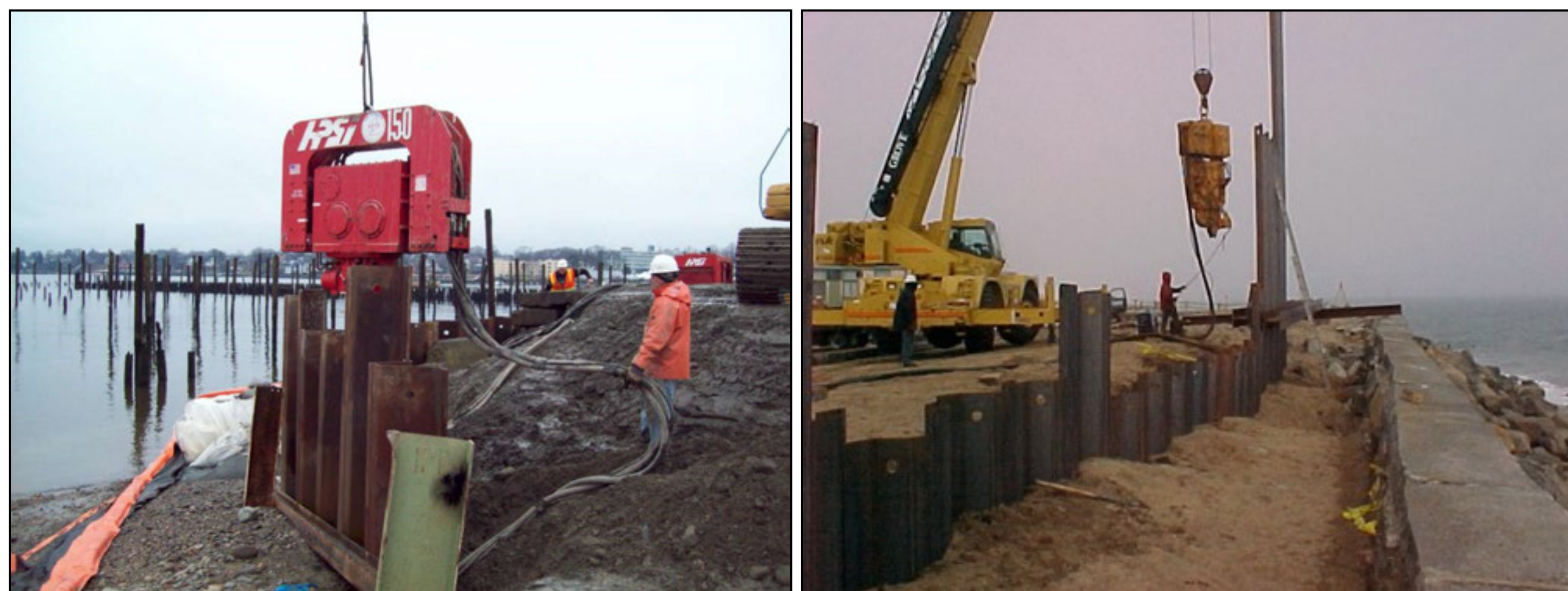
Construction of Barrier Wall - Sheet Pile Installation
