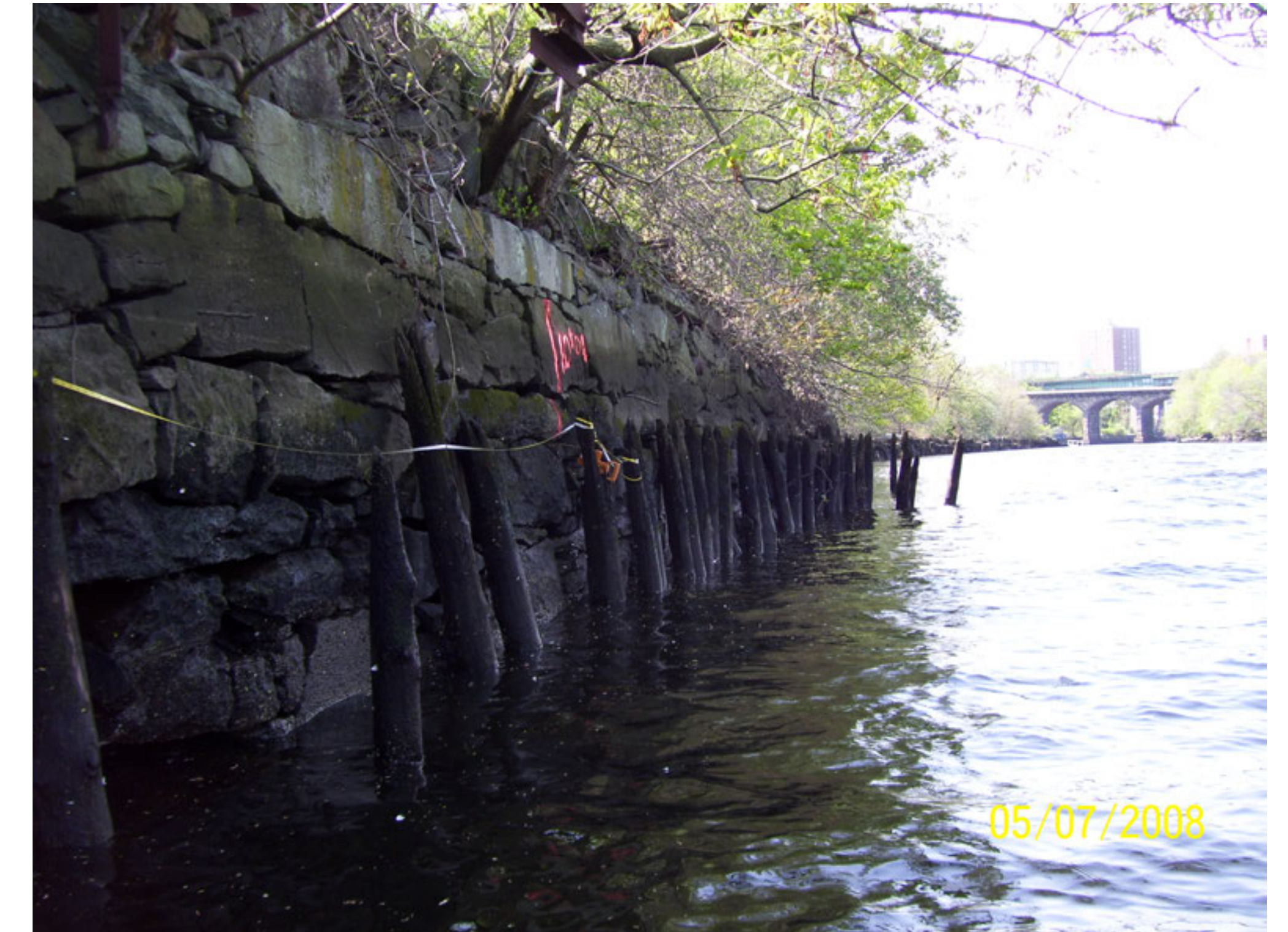
Granite Stone Block Walls Northern Portion of Site
