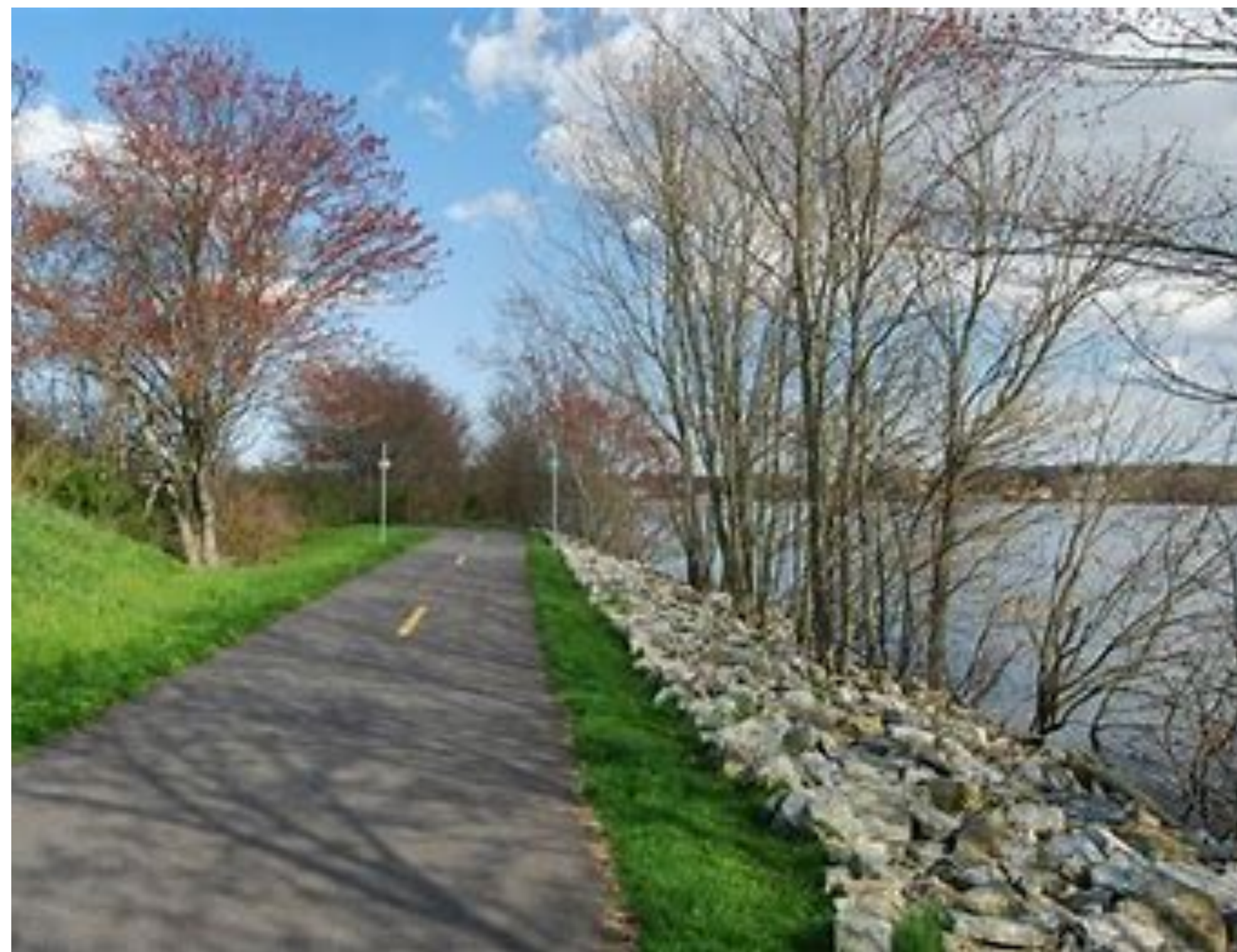
Example of Bike Path with Adjacent Revetment
