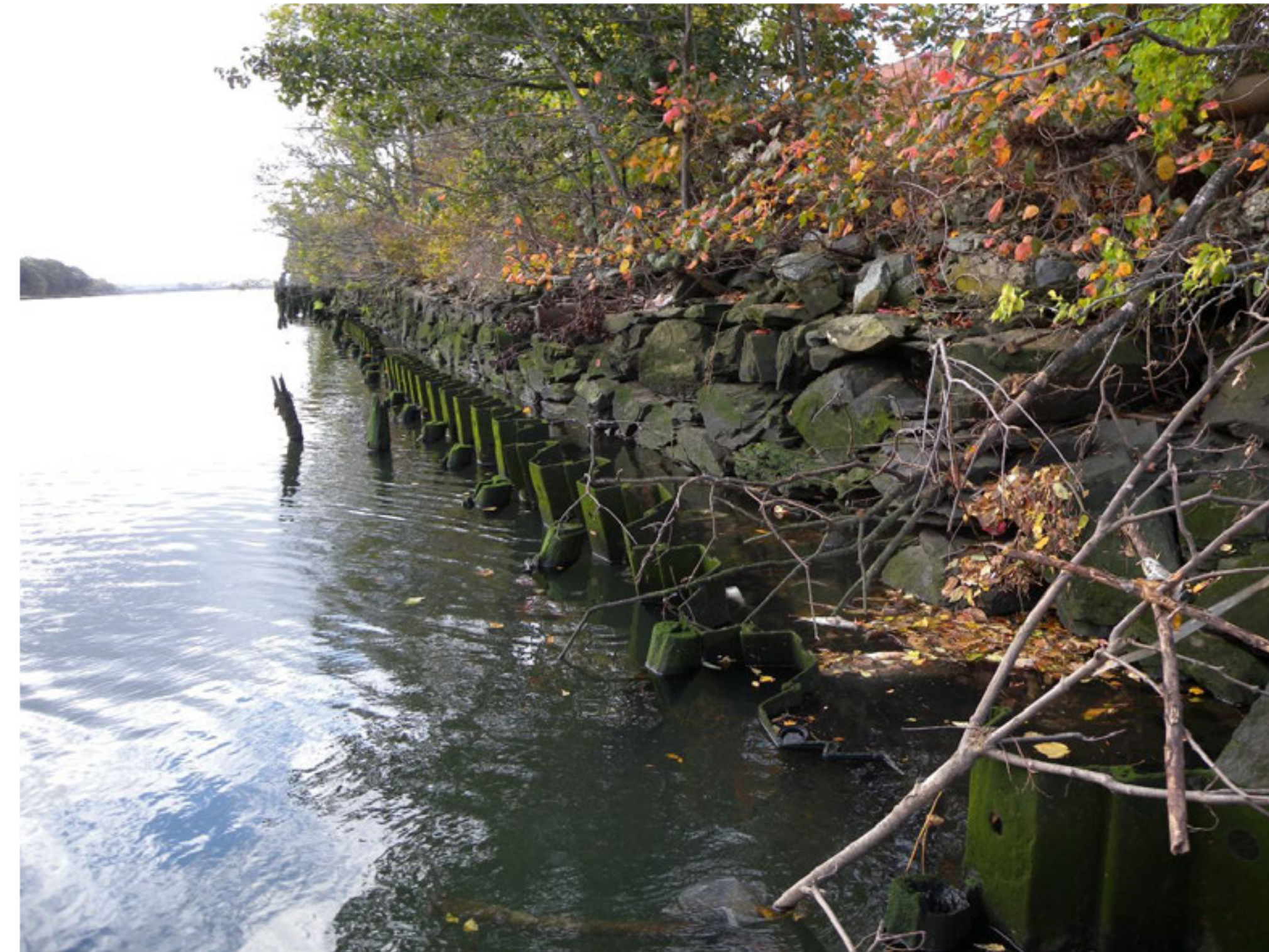
Granite Stone Block Wall and Steel Sheeting
