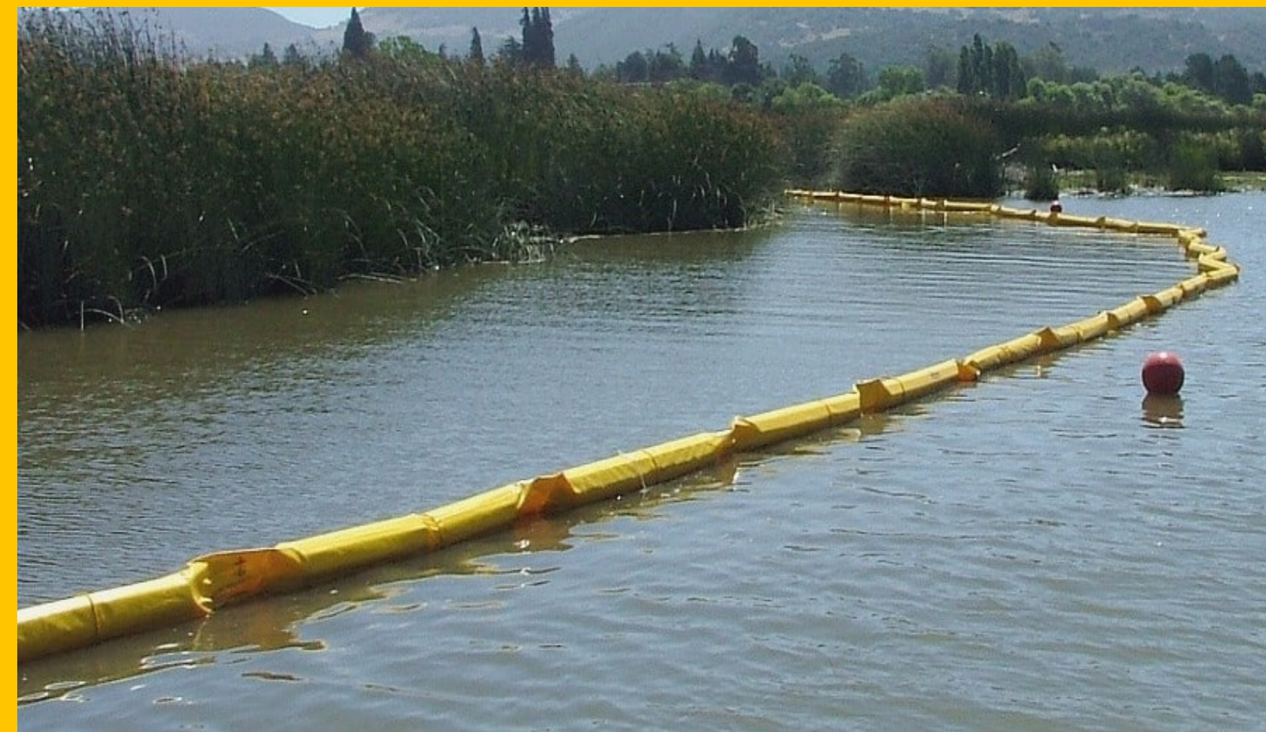
Turbidity Curtains Prevent Sediments From Migrating Away From Site
