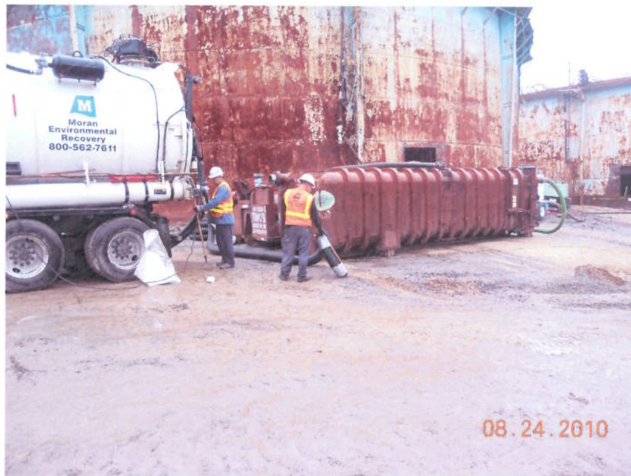
PHOTOGRAPH NO. 1 - Removal of visually impacted processed gravel with vector truck.
