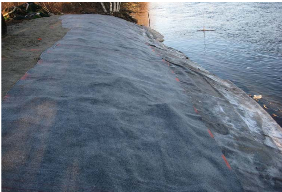
Photo No. 13 - Final RCM coverage
