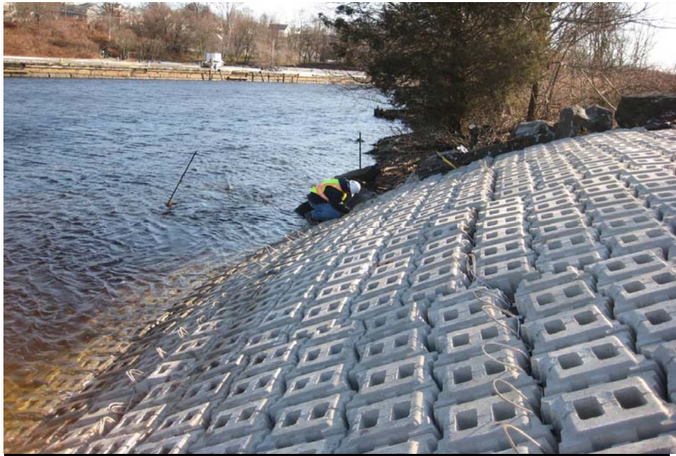
Photo No. 16 - Completed temporary cap, looking south
