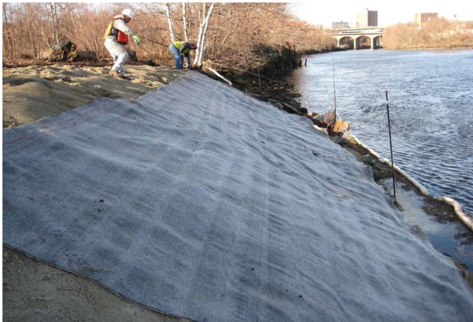
Photo No. 8 - Placement of RCM
