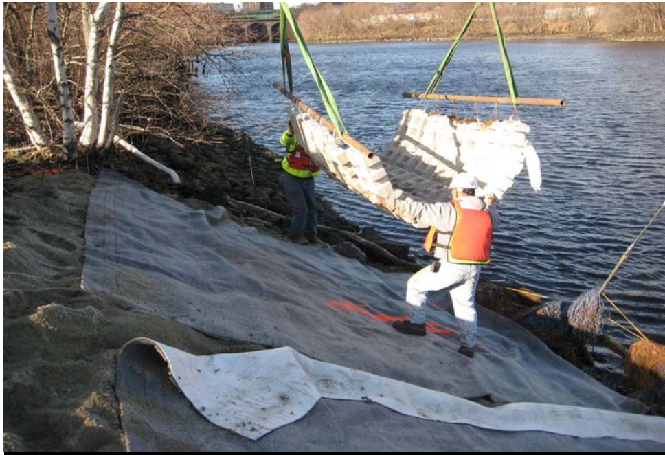
Photo No. 9 - Placement of armor mattress
