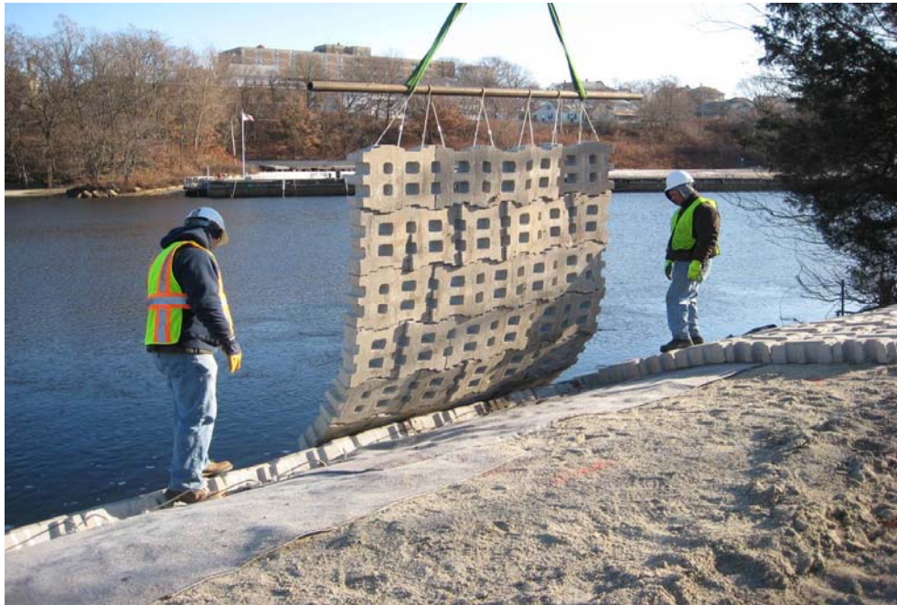
Photo No. 14 - Placement of final two rows of armor mattresses
