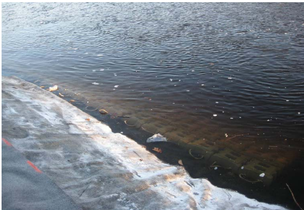
Photo No. 11 - Armor mattresses submerged at high tide the morning of December 17, 2009
