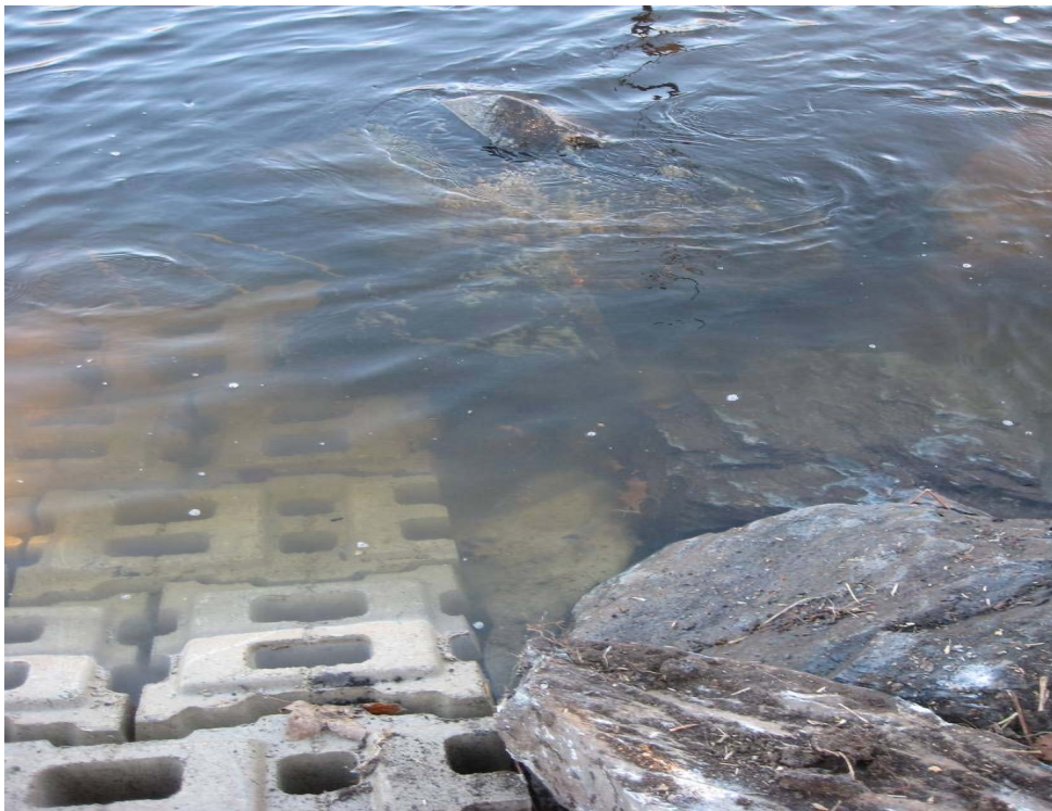
Photo No. 18 - Rocks covering exposure of RCM in southeast corner of temporary cap
