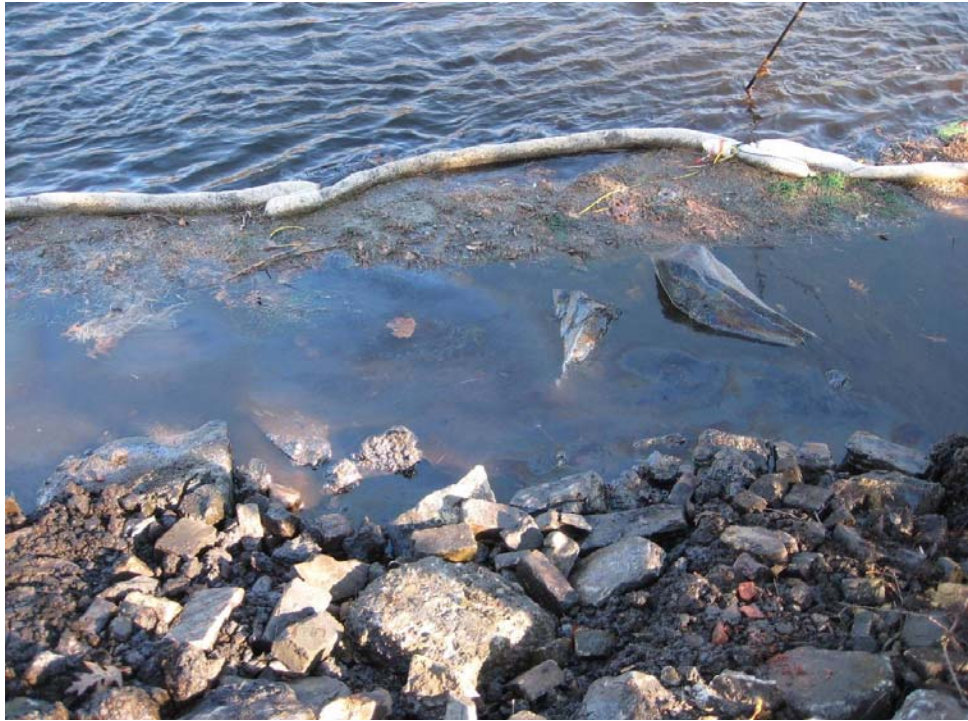
Photo No. 3 - Sheen emanating from voids following rock removal
