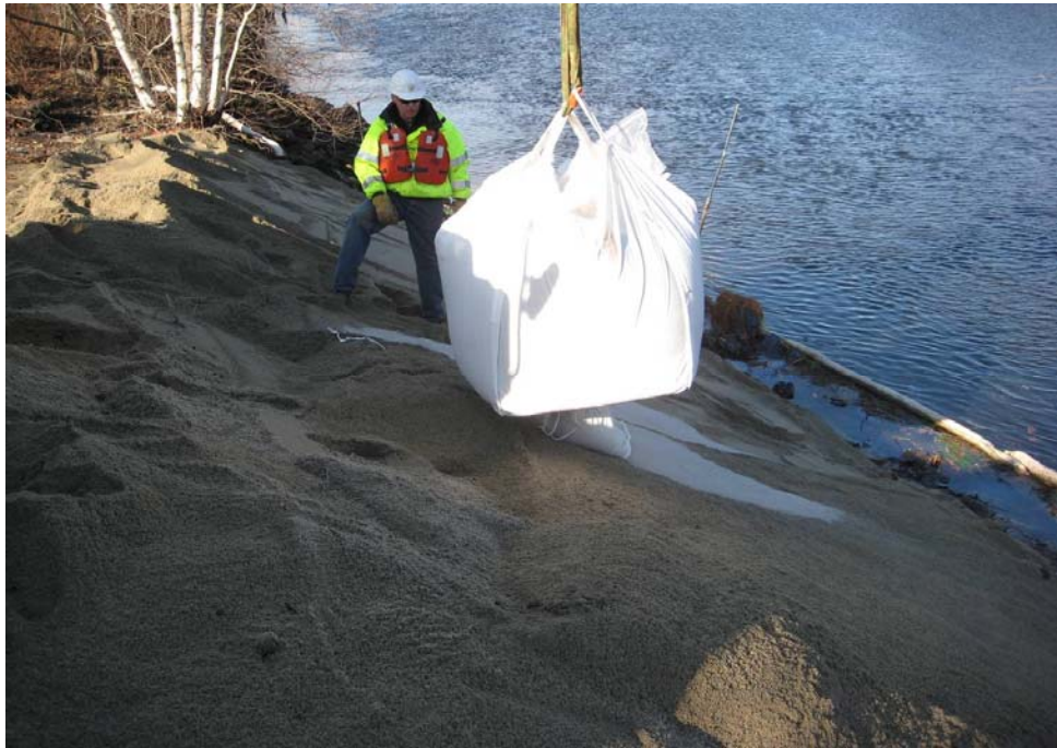
Photo No. 6 - Application of bulk organoclay to sand surface
