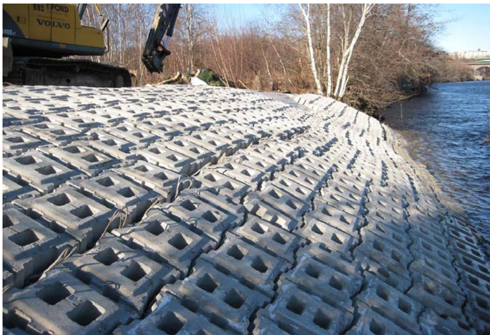
Photo No. 15 - Completed temporary cap, looking north
