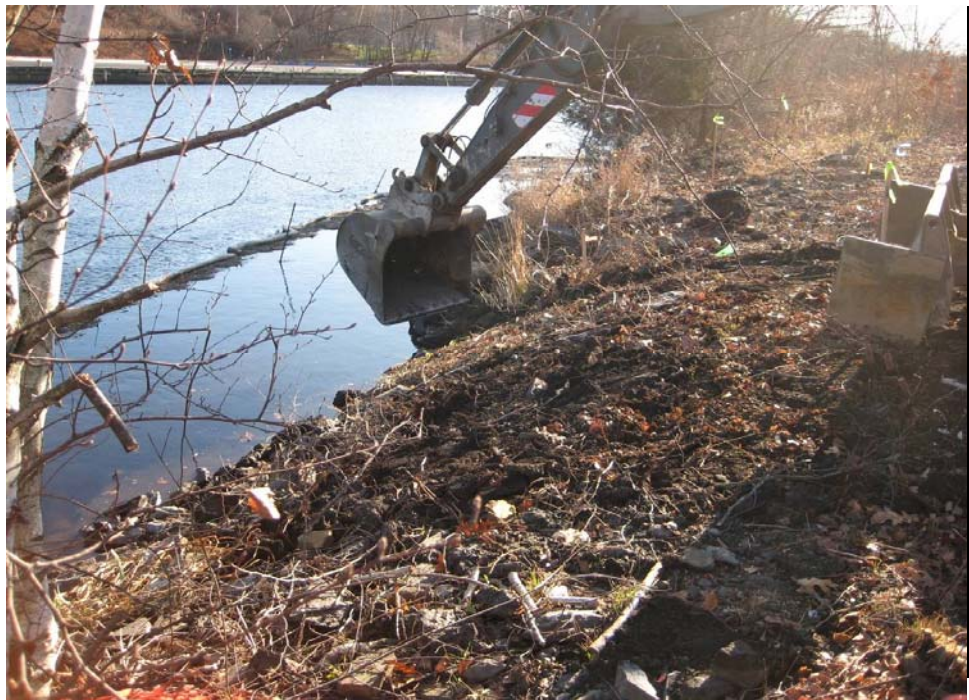
Photo No. 2 - Clearing and grading the riverbank
