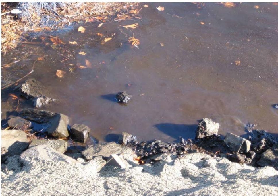
Photo No. 5 - Sheen emanating from toe of slope during bank work
