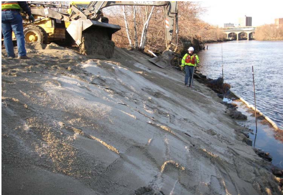
Photo No. 7 - Riverbank prior to RCM placement
