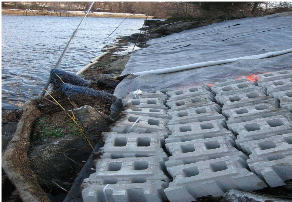
Photo No. 10 - RCM and armor mattress at northern corner showing minor design deviation where armor mattress could not be installed to low water line due to presence of obstructions, including boulders
