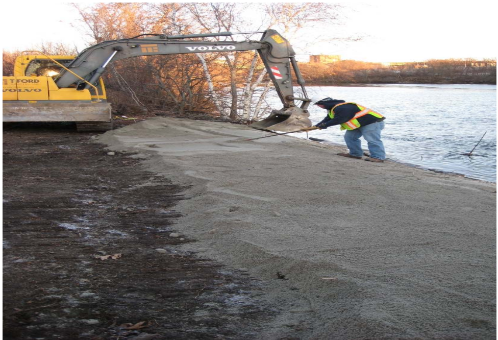
Photo No. 12 - Sand spreading to the top of the bank
