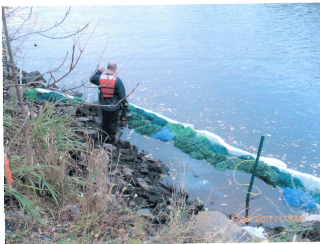
Photo 2: Containment Boom and Oil Snares Installed at Sheen Area
