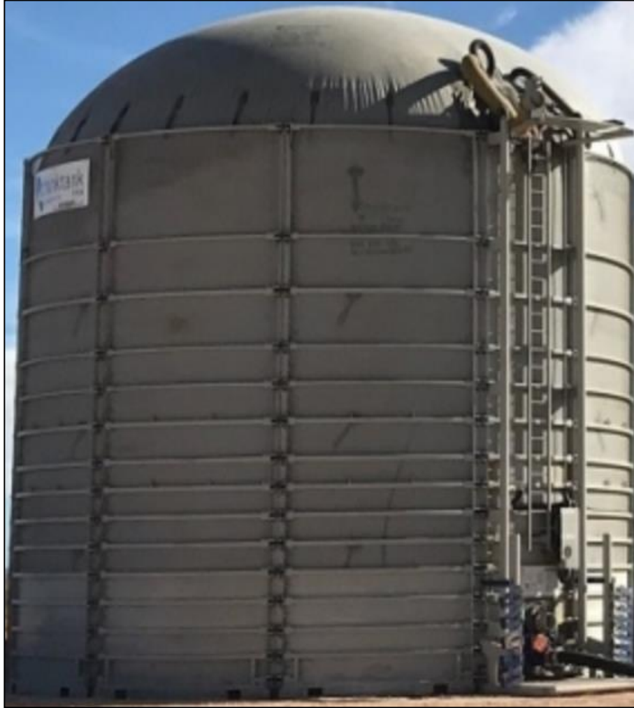
Figure 15. Picture of typical gas bladder
