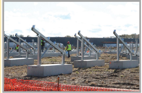
Above: Stanchions, used to support solar panels, line the site of the Kilvert Street solar park.
