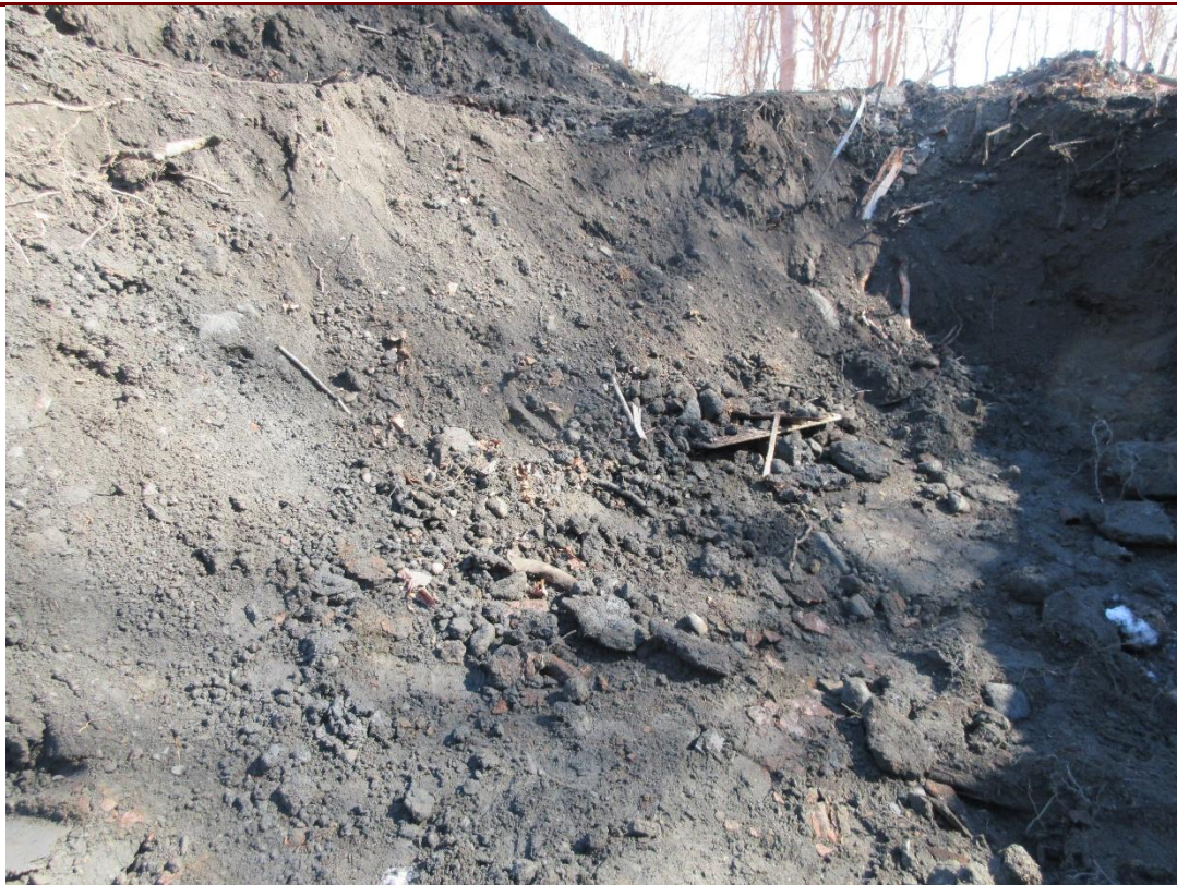
6. View of tank grave with no evidence of a petroleum release on March 13, 2019.
