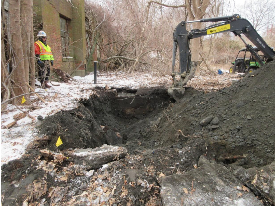
1. View of UST being uncovered by NRC on February 20, 2019.
