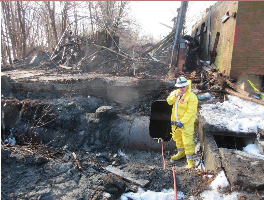
4. View of NRC personnel prepping to clean the tank on March 11, 2019.
