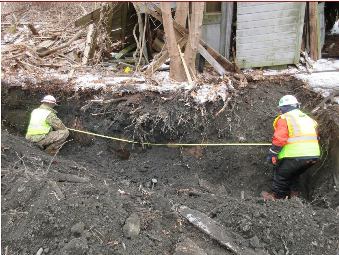
2. View of uncovered north side of the UST on February 20, 2019.
