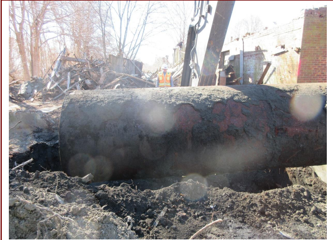
7. View of bottom of tank with no evidence of corrosion or holes.
