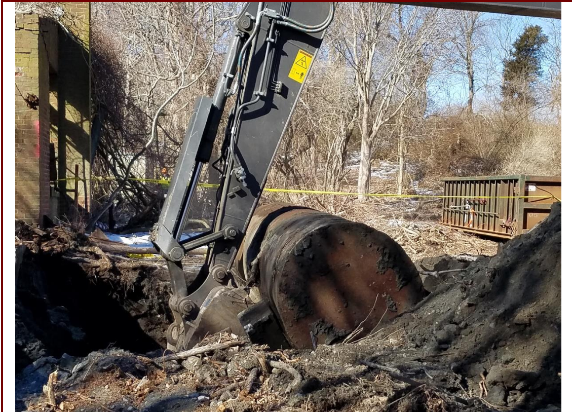
5. View of EnviroVantage unearthing tank on March 13, 2019.
