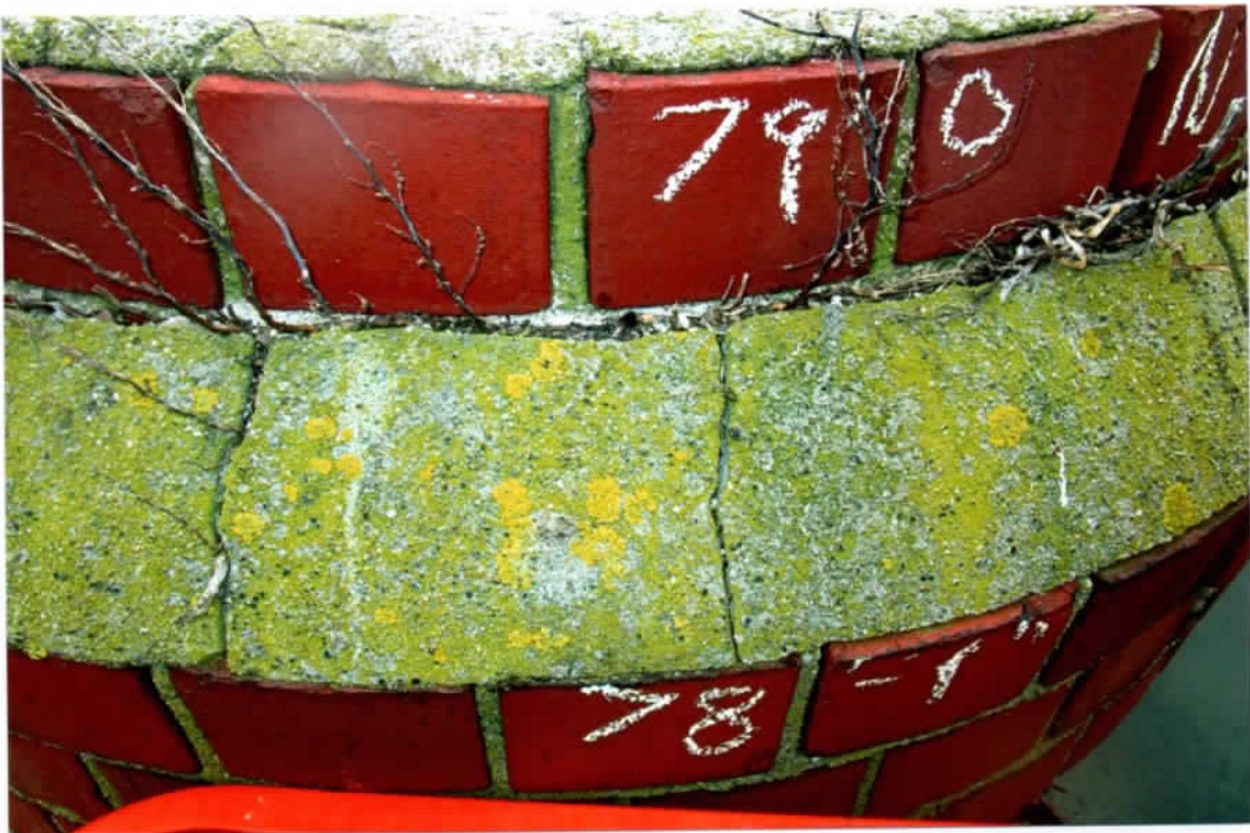
Photo 16. Close-up of cracked and loose sections of the water table (northeast side).
