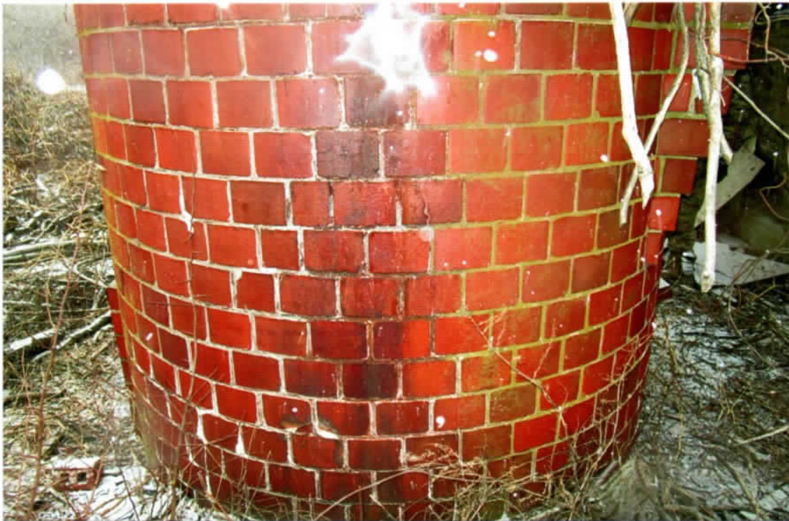
Photo 42. Fair exterior condition of the south side in the 5' above grade. A few random deteriorate and open mortar joints were seen in this region below the entering duct.
