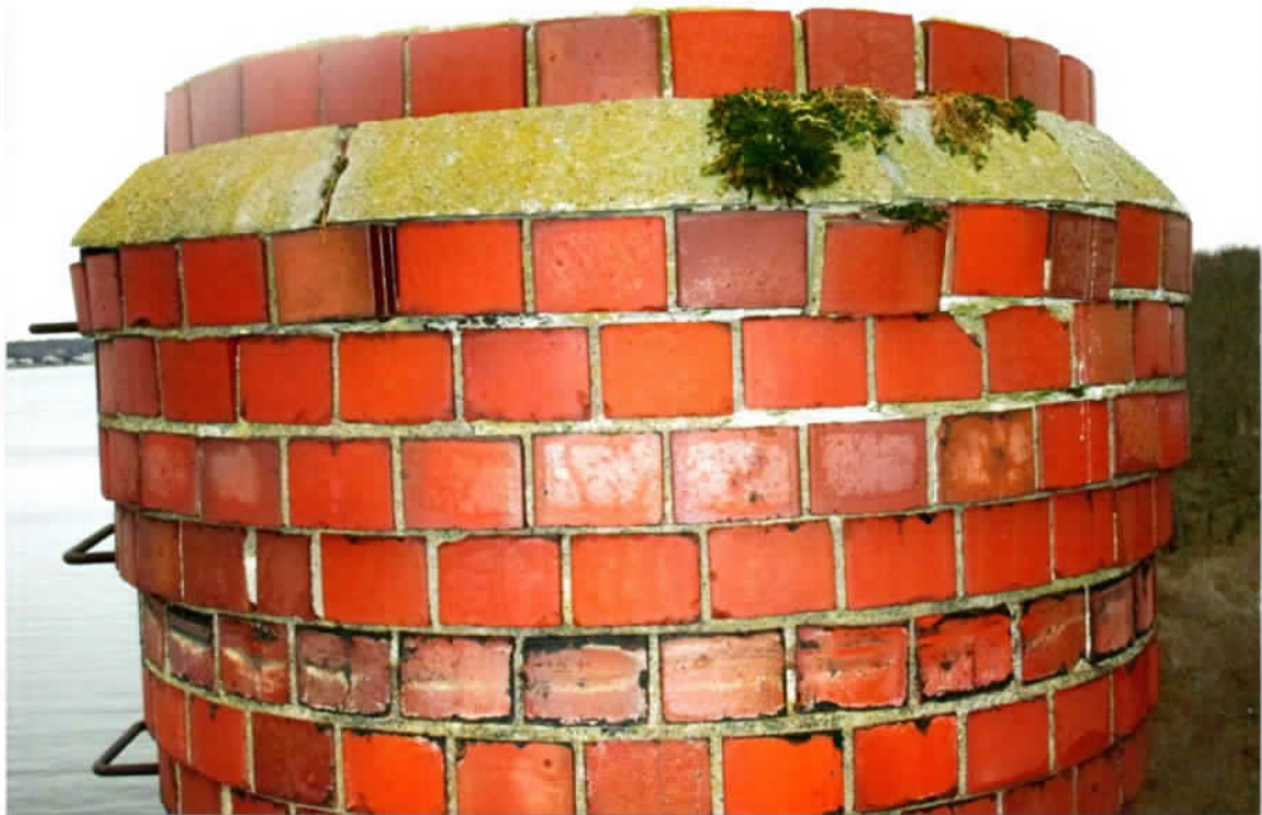
Photo 19. Poor condition of the upper 4' of the south side. Several loose and unstable bricks were seen below the water table.
