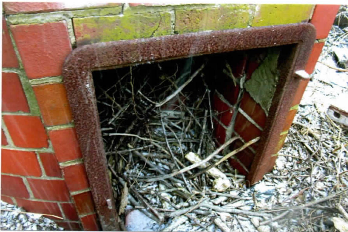
Photo 48. Deteriorated and pitted frame of the original cleanout opening. Note the accumulated brush and debris on the interior.
