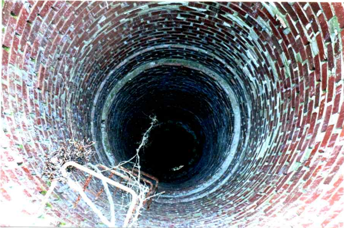
Photo 11. Fair interior condition between the 60' and 50' levels. Mortar joints were only slightly recessed in this region.
