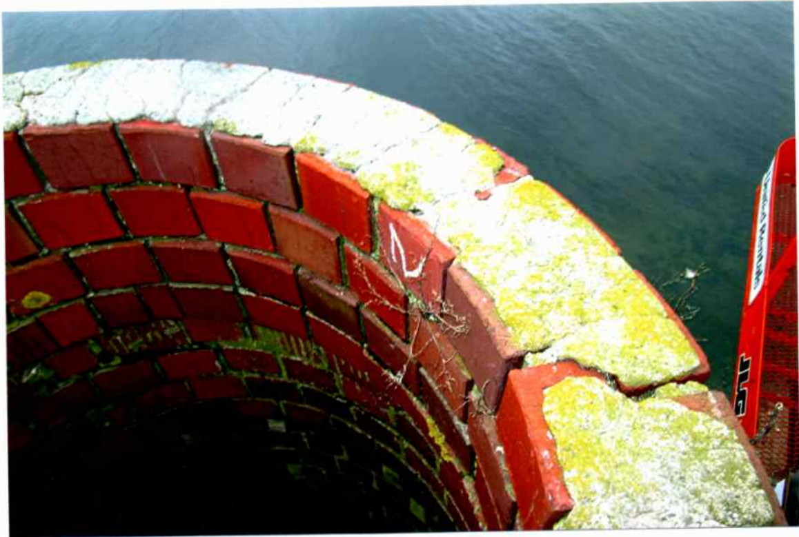
Photo 3. Poor condition of the remaining cement cap atop the chimney (north side).
