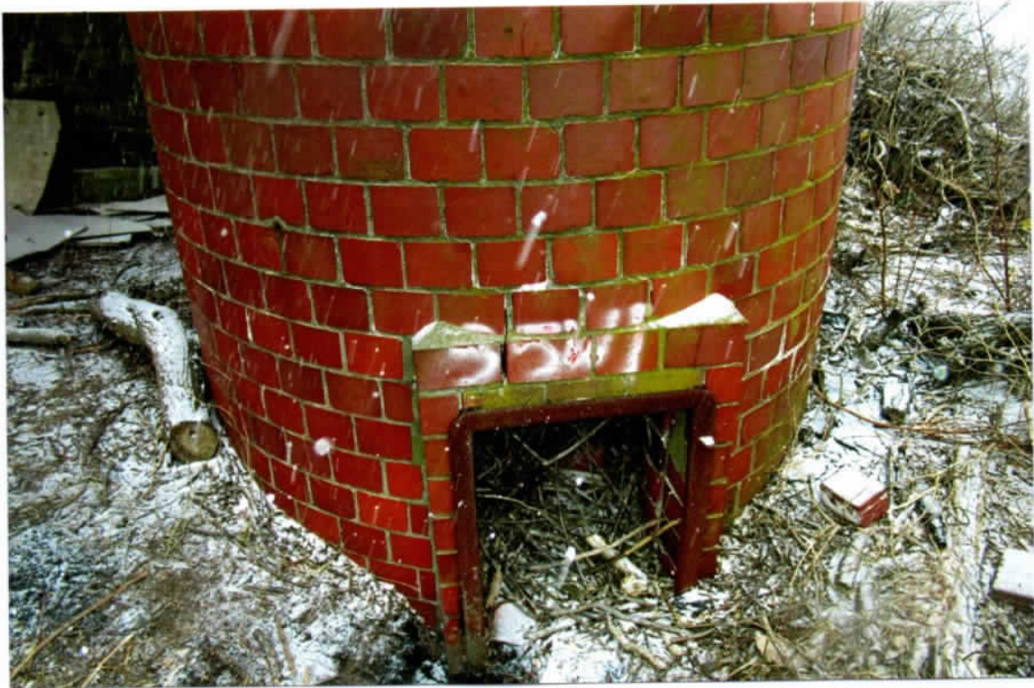
Photo 47. Fair exterior condition of the lower north side local to the cleanout opening. A few open mortar joints were identified. Note the missing cleanout door.
