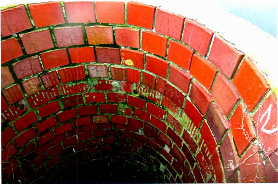
Photo 9. Fair interior condition of the upper elevations (northwest side). No concerns were seen with brick faces but mortar joints were recessed up to \frac{3}{4} " near the top.
