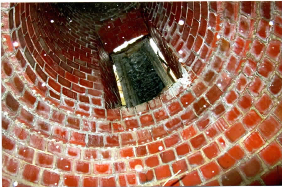
Photo 50. Overall good interior condition of the inner liner wall below to the duct opening. No obvious concerns were seen with the lower structural wall or corbelled support of the liner.
