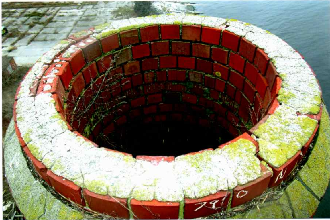
Photo 1. Poor condition of the remaining cement cap atop the chimney. Note the deteriorated and dislodged areas of the thin layer of material.
