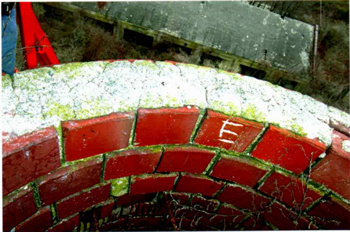
Photo 5. Poor condition of the remaining cement cap atop the chimney (east side).
