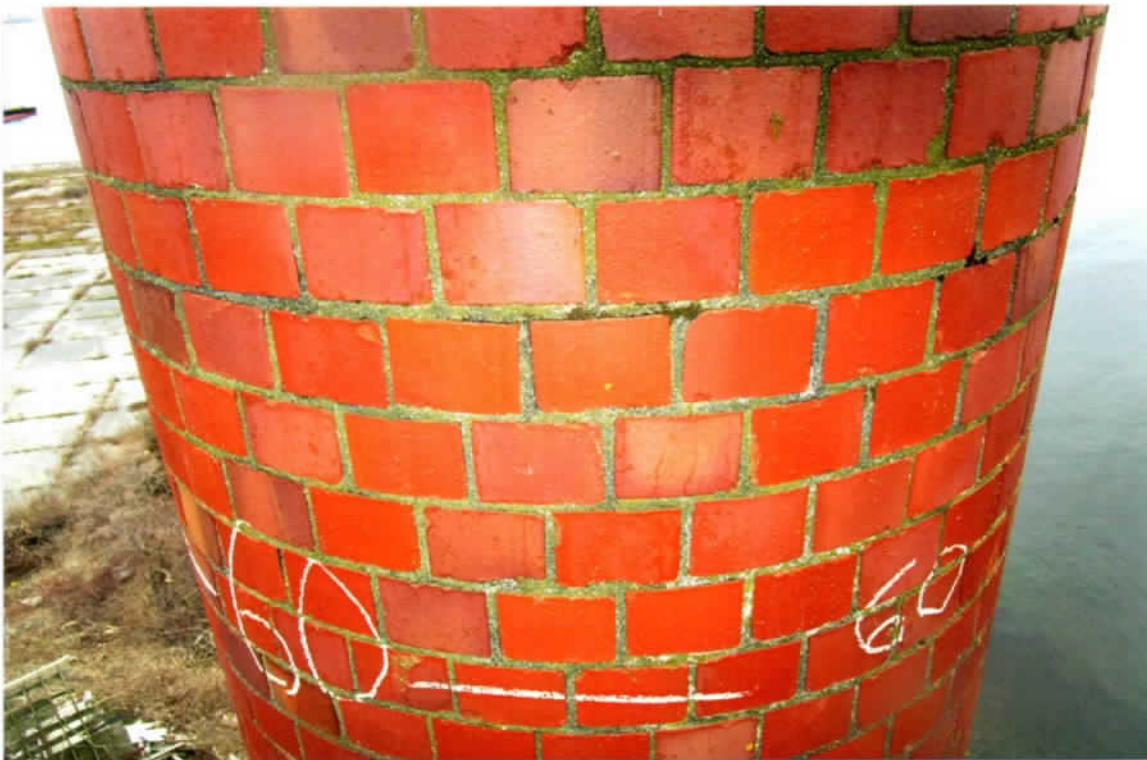
Photo 30. Fair exterior condition of the northeast side local to the 60' levels. Mortar joints were only slightly recessed in this region.
