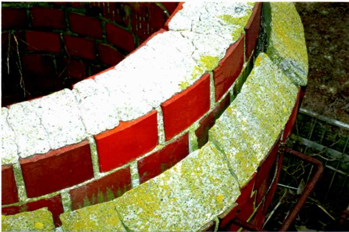
Photo 14. Close-up of loose and unstable sections of the water table (west side). Sections on this side were in danger of dislodging.
