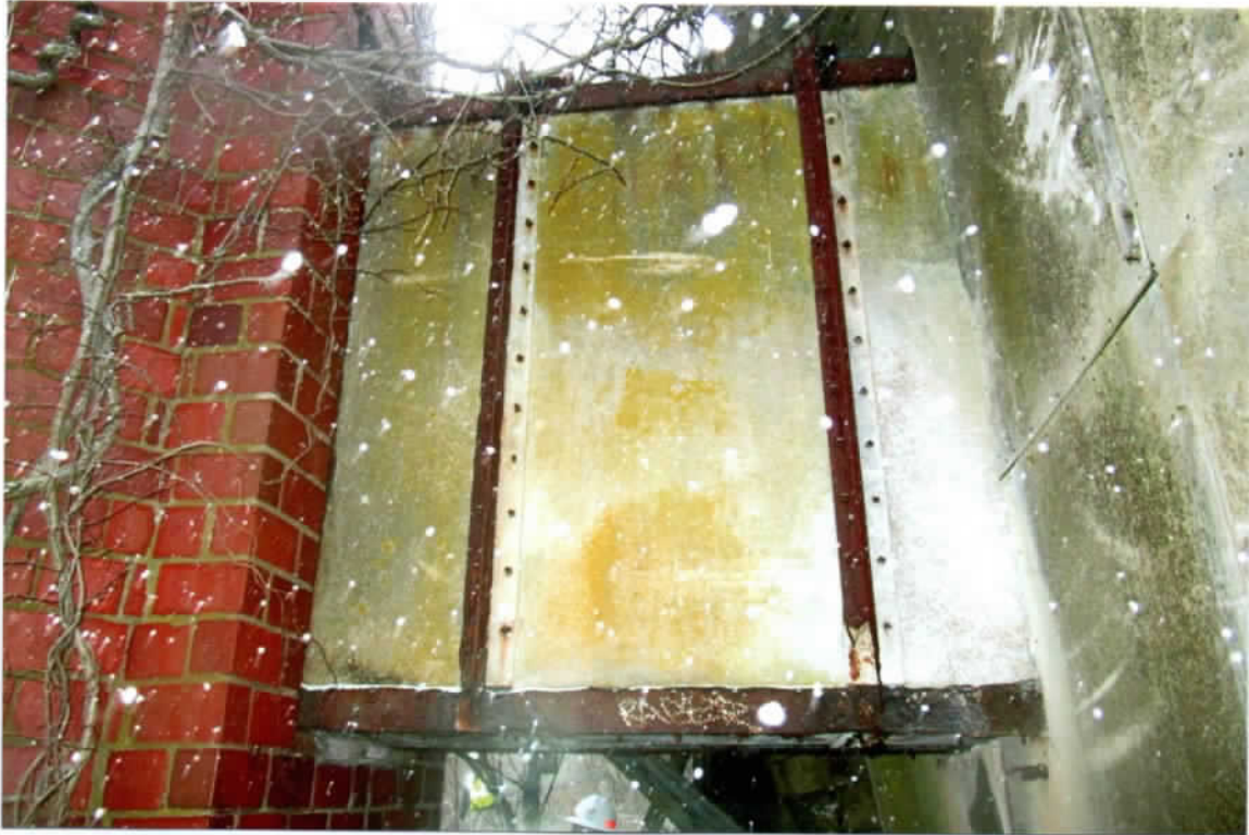
Photo 41. Poor condition of the boiler duct extending from the boiler house to the chimney. The steel angle frames were severely eroded. The duct was not in danger of collapsing.
