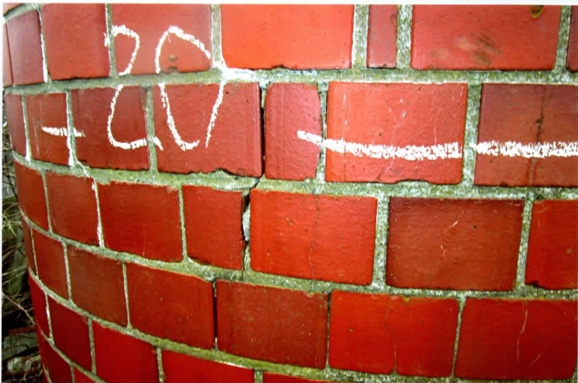
Photo 38. Fair condition of the east side near the 20' level. Note the open joints along the three courses. No cracked bricks were identified.
