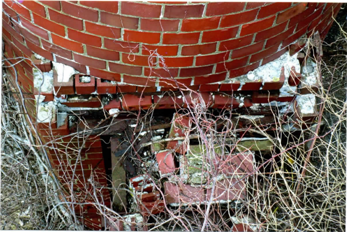
Photo 39. Very poor condition of the extended wall and lintels above the boiler duct opening. Numerous dislodged bricks were identified, and the condition of the lintel beams was poor.
