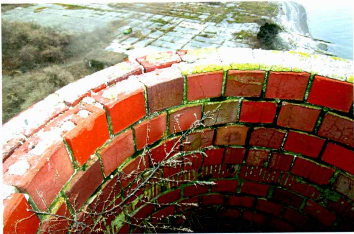
Photo 4. Very poor condition of the remaining cement cap atop the chimney (south side). Note the region where the cement has completely dislodged.
