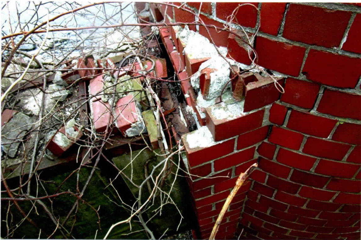
Photo 40. Very poor condition of the extended wall and lintels above the boiler duct opening. Numerous dislodged bricks were identified, and the condition of the lintel beams was poor.
