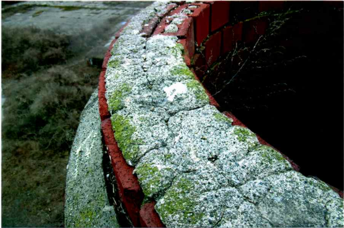
Photo 7. Close-up of the remaining deteriorated cement cap atop the chimney.
