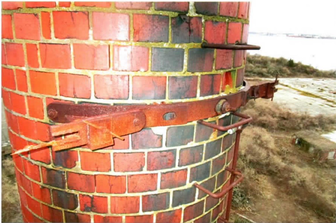
Photo 27. Fair condition of the anchored steel bracket at the 71'-6" level (northwest side). The bracket was deteriorated but secure to the wall.
