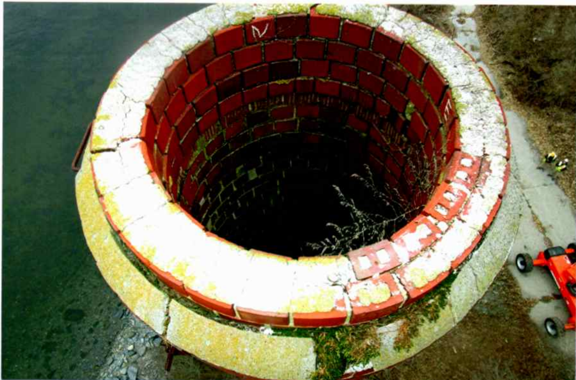
Photo 2. Poor condition of the remaining cement cap atop the chimney.
