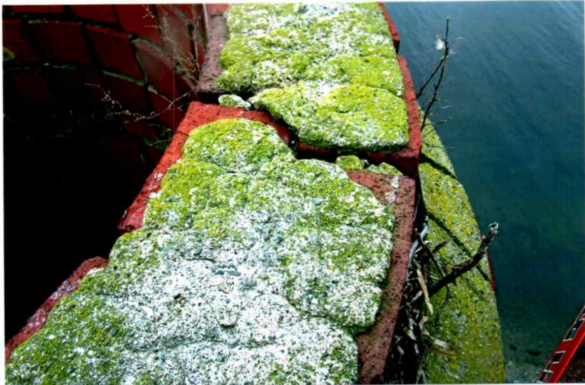
Photo 8. Close-up of the remaining deteriorated cement cap atop the chimney.
