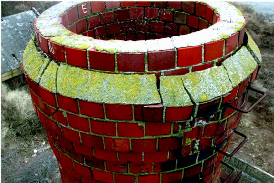
Photo 13. Poor exterior condition of the upper elevations (northwest side). Note the cracked water table (cement wash). Several bricks were in danger of dislodging.
