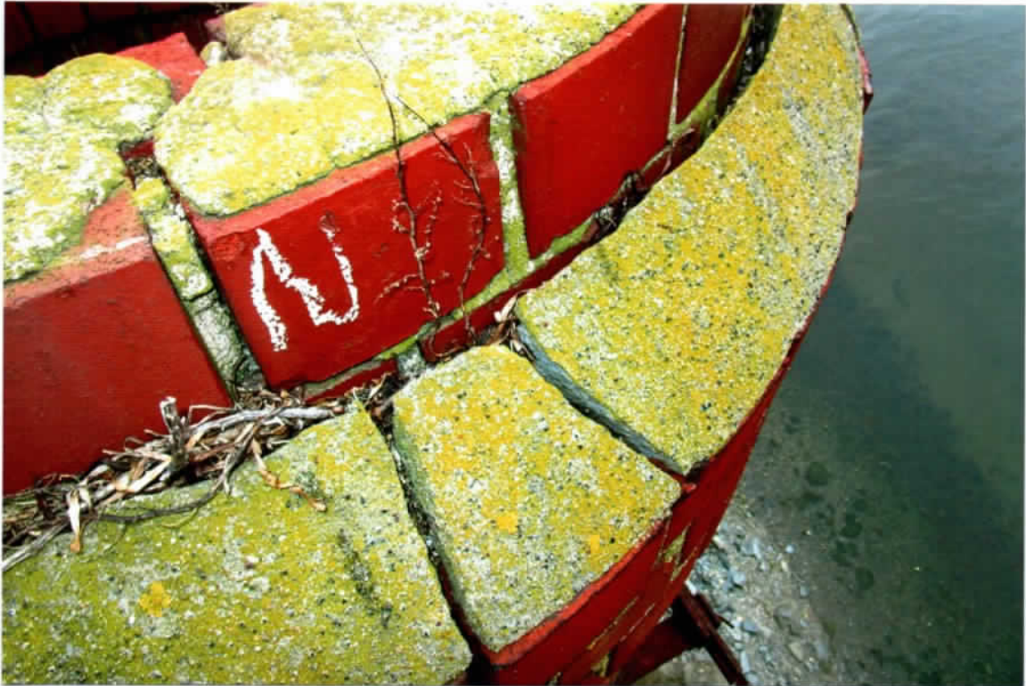
Photo 15. Close-up of cracked and loose sections of the water table (north side).
