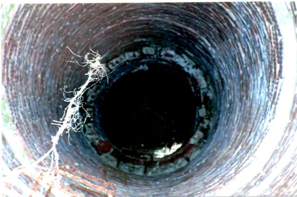
Photo 12. Poor condition along the top of the inner liner wall near the 29' level. Numerous loose and unstable bricks were seen along the top of the inner liner wall.
