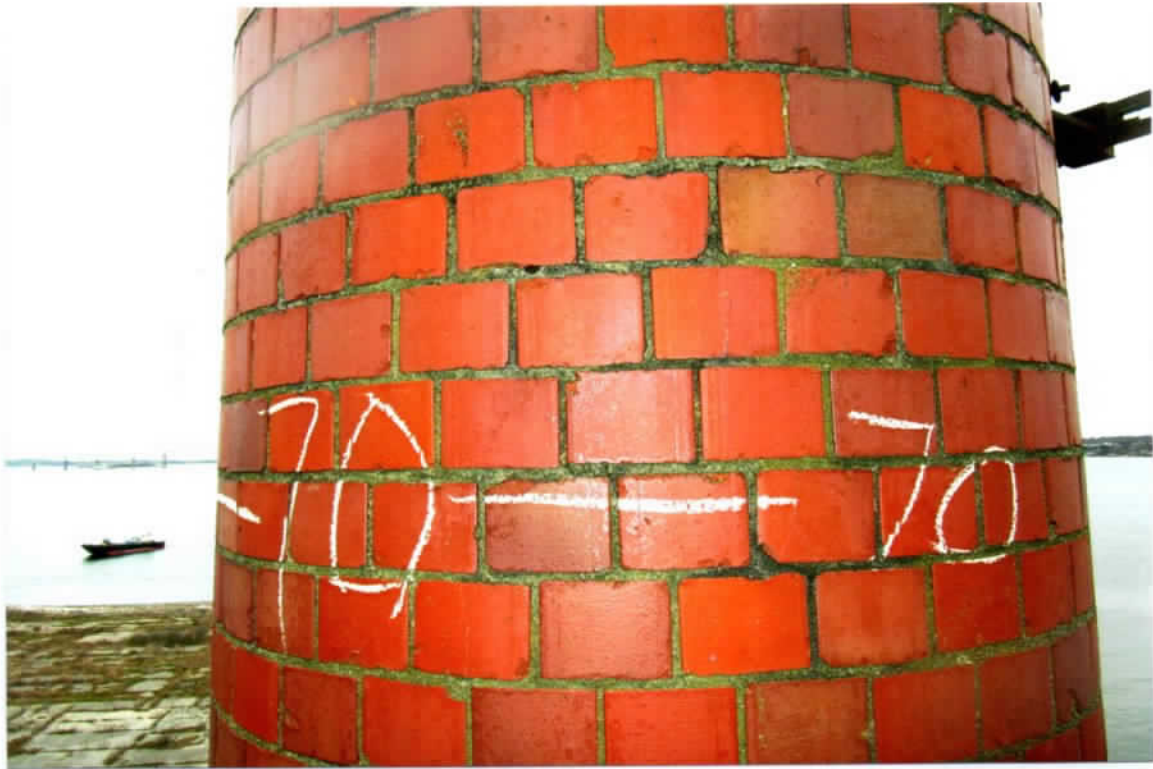
Photo 29. Fair exterior condition of the northeast side local to the 70' levels. Mortar joints were only slightly recessed in this region.
