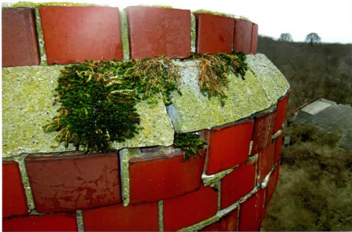
Photo 21. Close-up of unstable bricks and sections of the water table (southeast side). The one brick and small section of cement water table were removed during the inspection.
