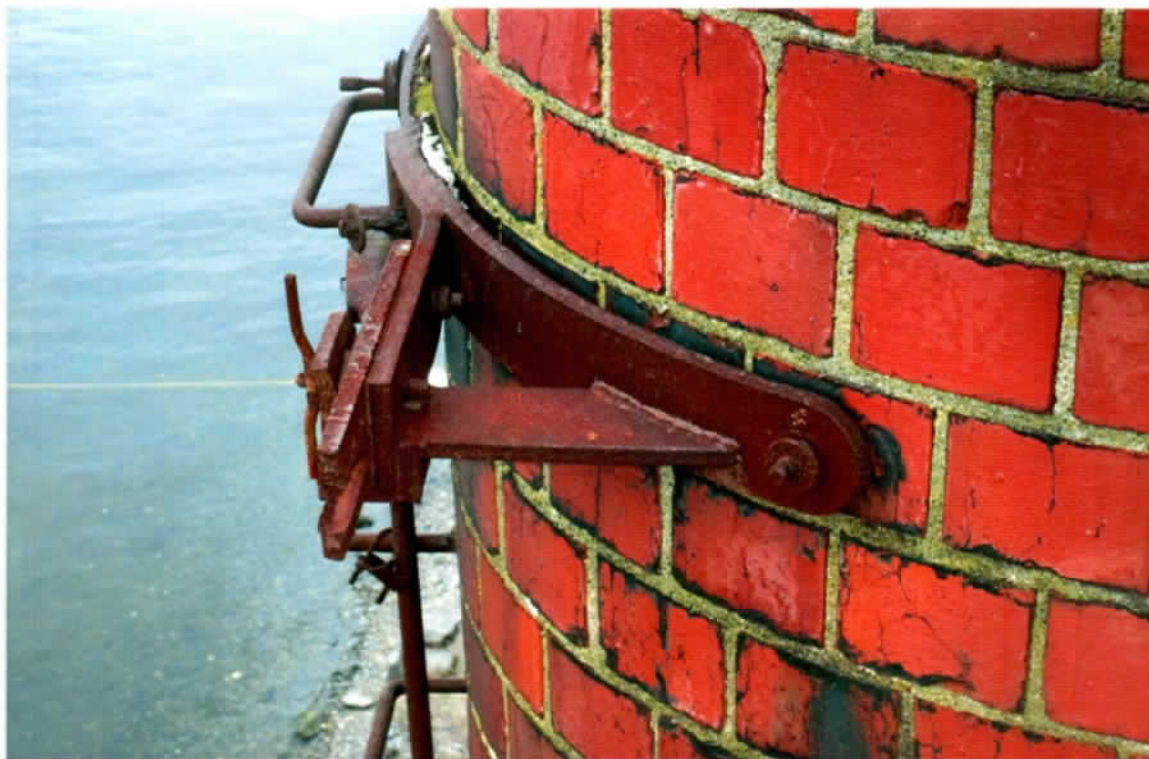
Photo 28. Fair condition of the anchored steel bracket at the 71'-6" level (southwest side). The bracket was deteriorated but secure to the wall.
