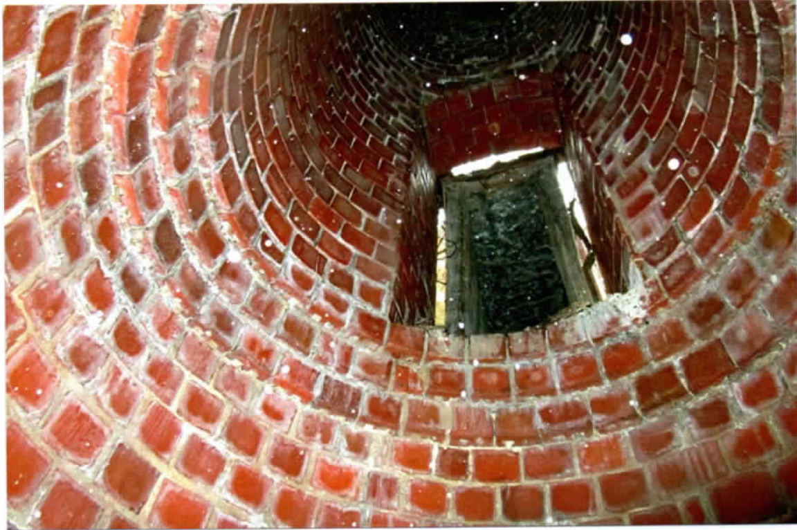
Photo 49. Overall good interior condition of the inner liner wall local to the duct opening. No obvious concerns were seen with the lower structural wall or corbelled support of the liner.
