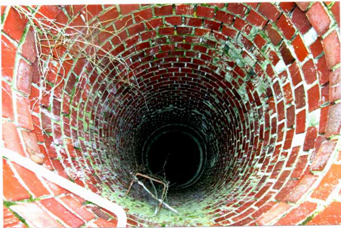
Photo 10. Fair interior condition of the upper elevations looking down from the top. No concerns were seen with brick faces. Local areas of mortar joints were recessed \frac{3}{4} " to 1".
