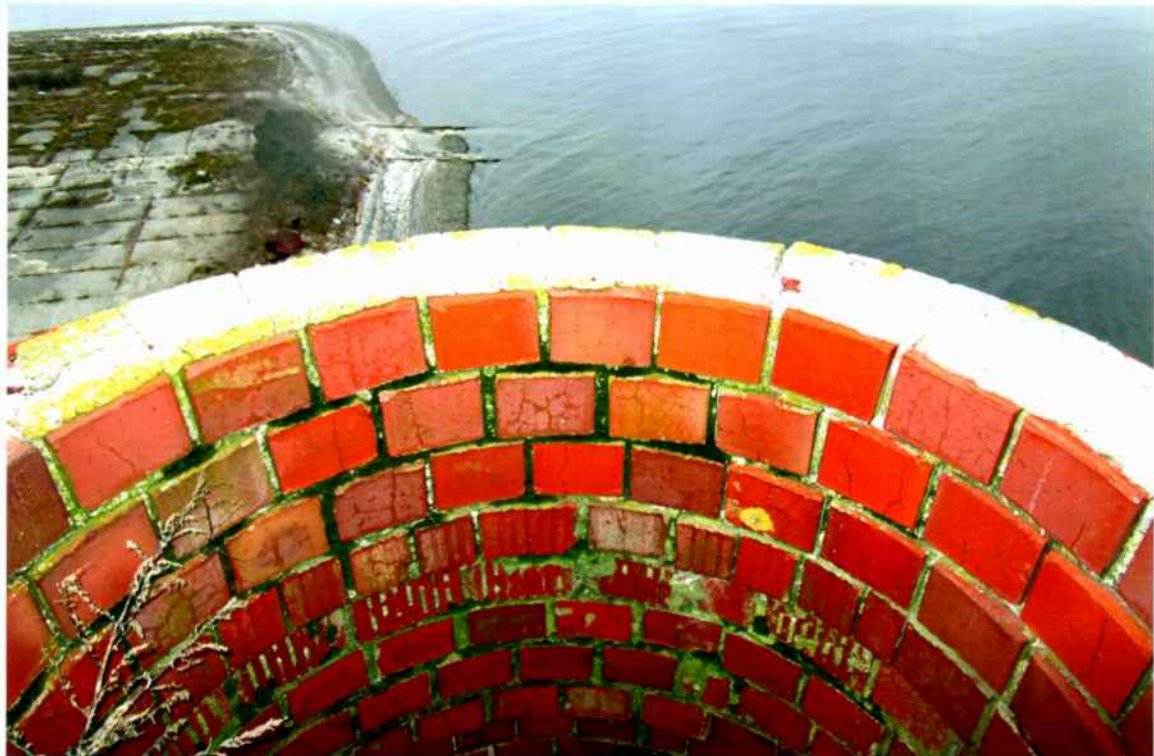
Photo 6. Poor condition of the remaining cement cap atop the chimney (west side).
