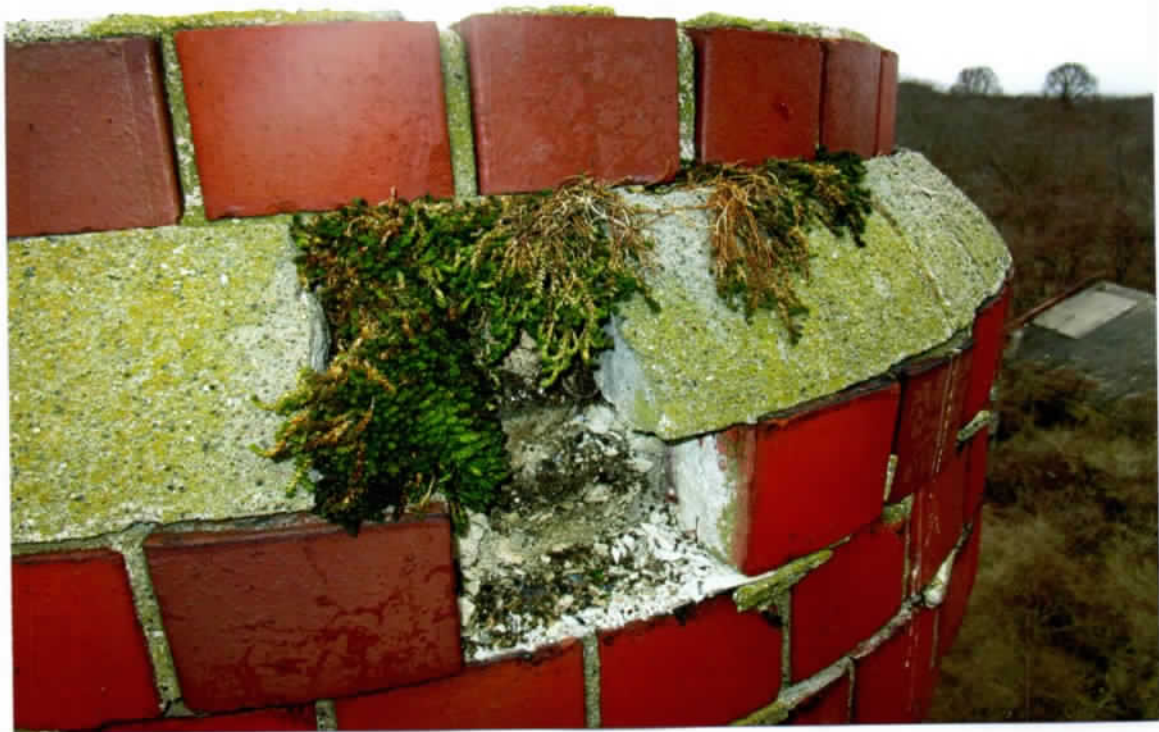
Photo 22. Picture showing the upper southeast side after removing the one brick and small section of cement water table.
