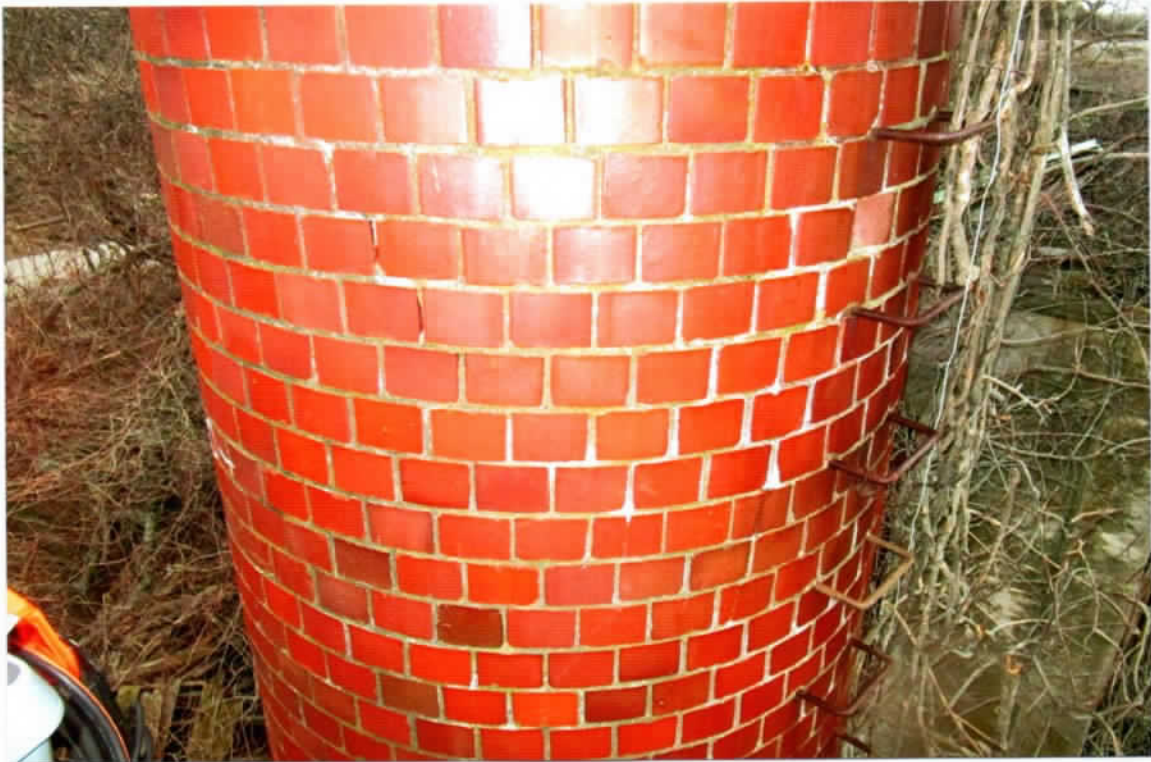
Photo 36. Fair exterior condition of the southwest side near the 20' level. A few random deteriorate and open mortar joints were seen in this region.
