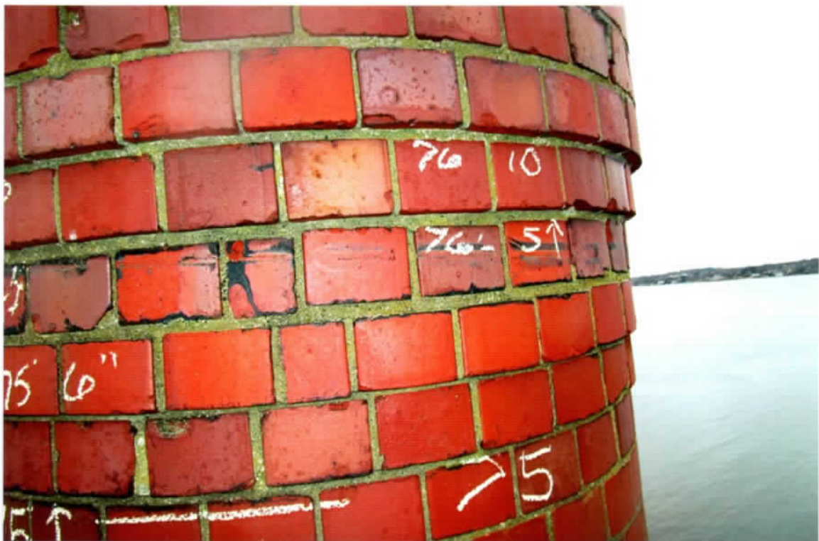
Photo 24. Fair condition of the northeast side between the 77' and 75' levels. No obvious or immediate concerns were seen in this region.
